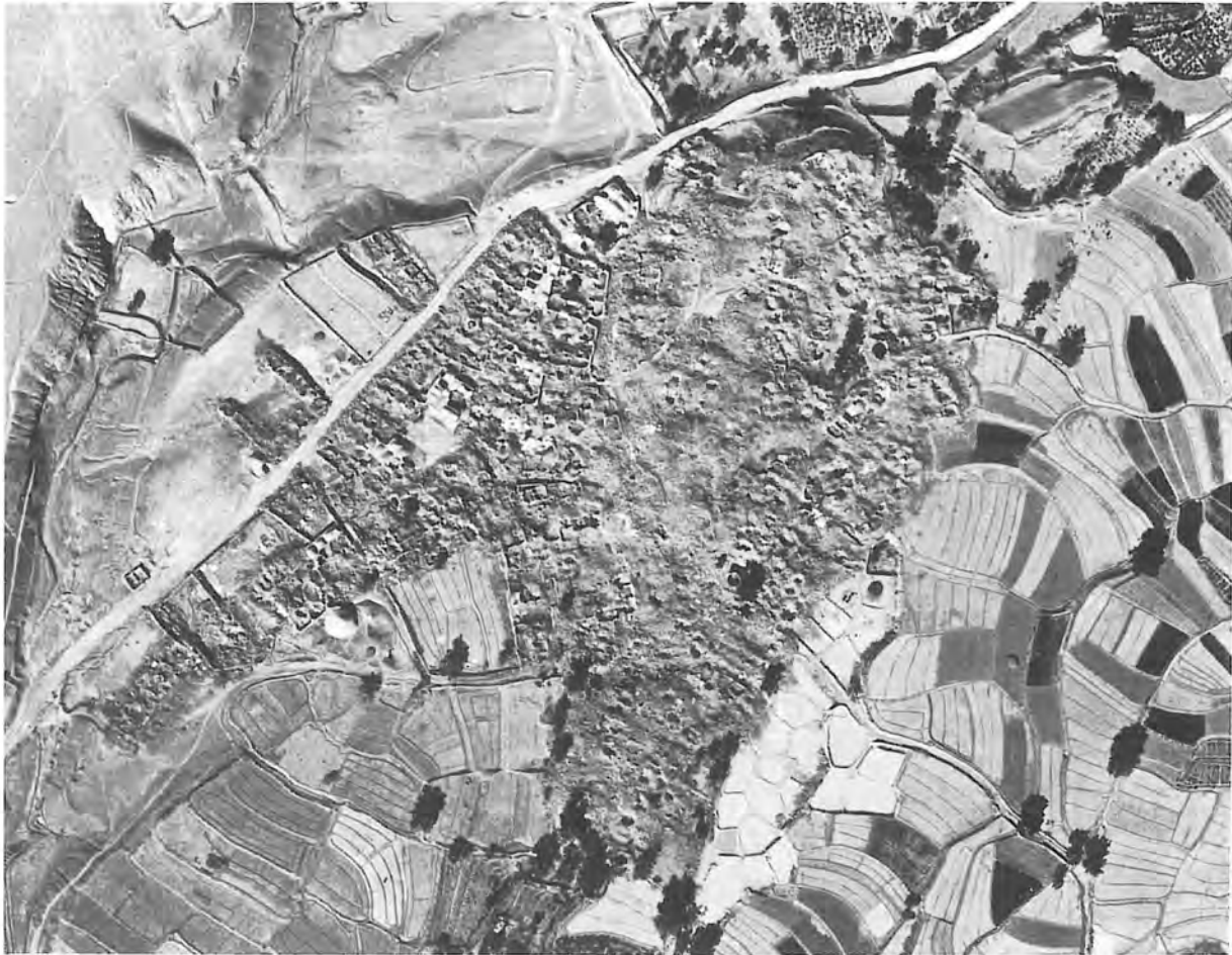
Plate 2(b). Another victim of the Dasht-i Biyaz earthquake: no domes remain intact.
