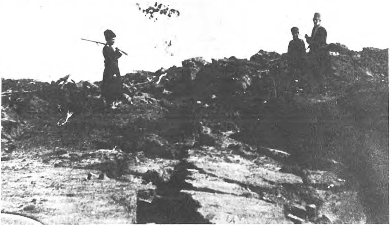
Plate 10. Fault break of Sandargan associated with the 1909 earthquake in Silakhur. Photograph taken by the Russian mission, members of which are seen in the background.
