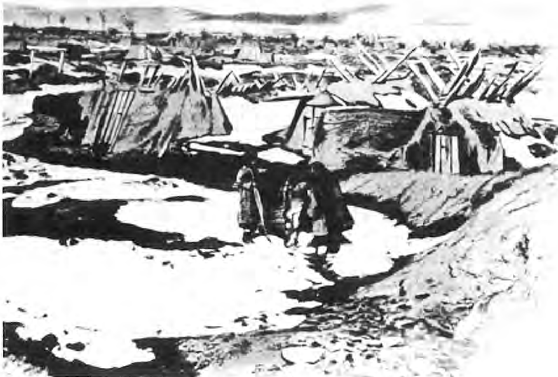
Plate 27. A-shaped shelters put up in Quchan after the earthquakes of 1893 and 1895. Other views of this type of construction are shown in Huntington (1905: 236) and MacGregor (1879: 85).
