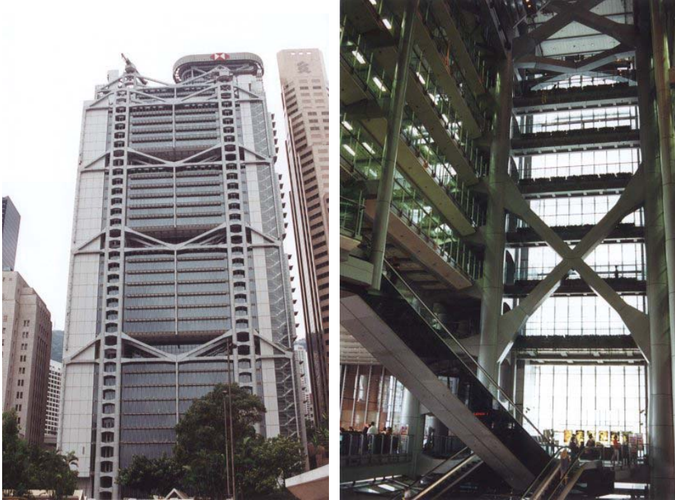
Fig. 3.24 HSBC headquarters in Hong Kong.
