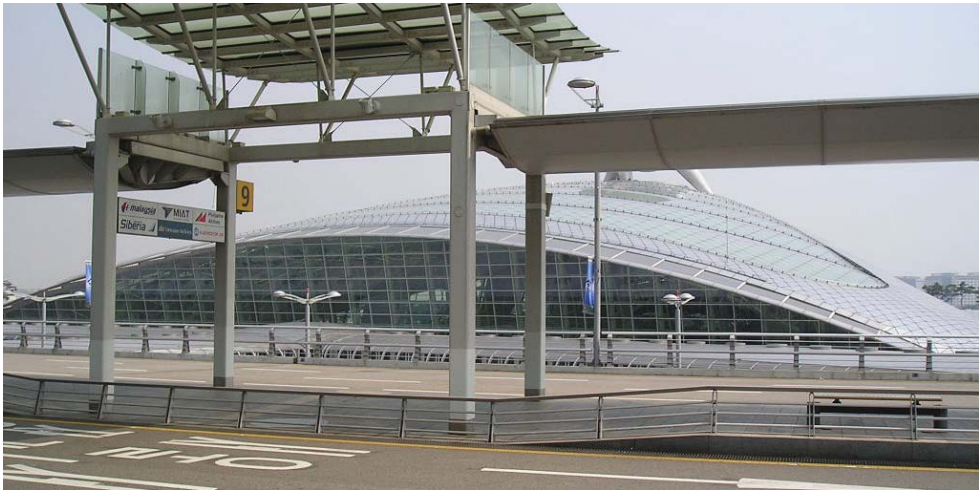
Fig. 8.3 Latticed shell structures: Incheon airport Korea.
