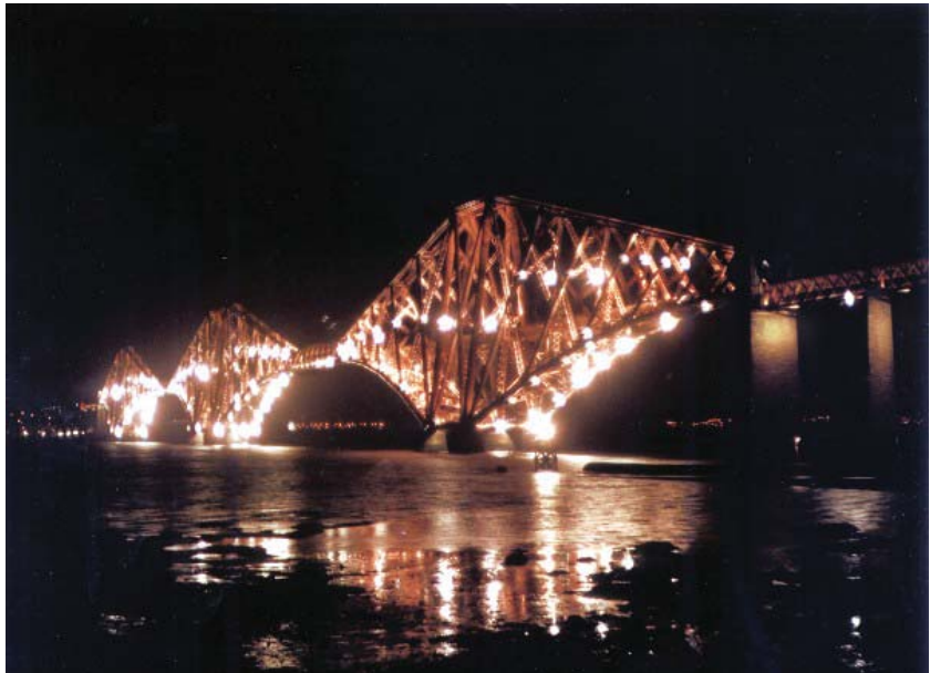
Fig. 9.3 Forth Bridge. Photo from Structurae: International Database for Structural Engineering, courtesy of Wilhelm Ernst & Sohn Verlag.
