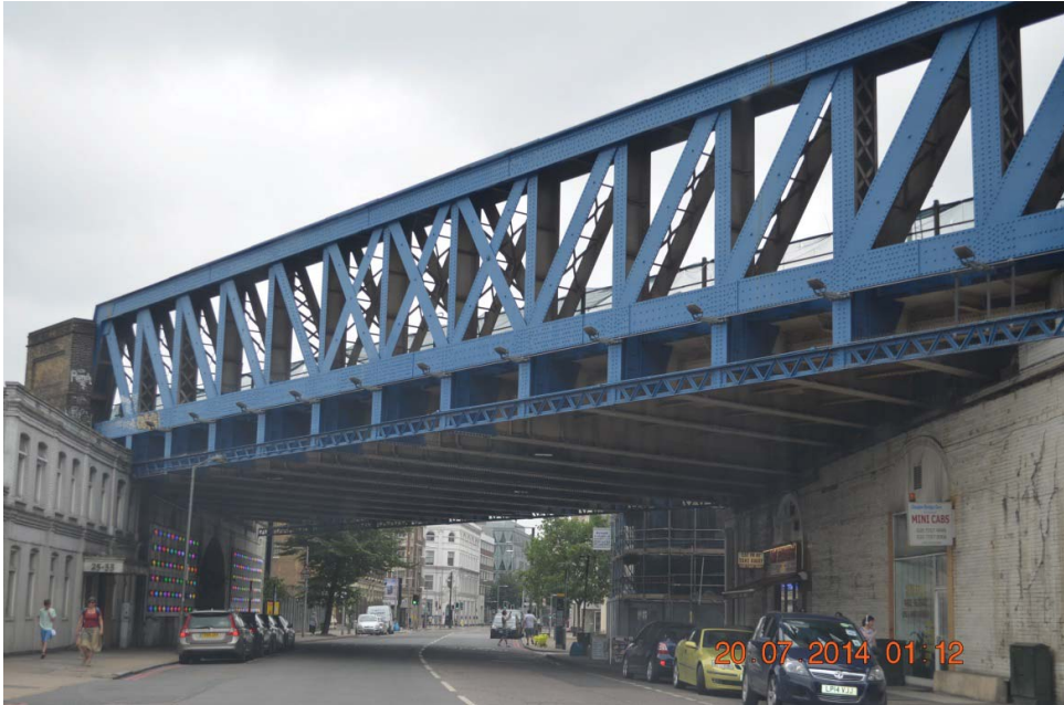
Fig. 9.1 Illustration of a truss beam bridge in London.
