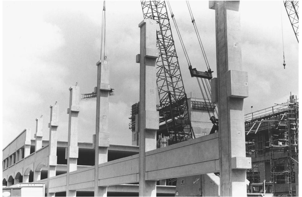
FIGURE 19.22 Precast parking garage at Cornell University. ( Photo- graph by Arthur H. Nilson. )
