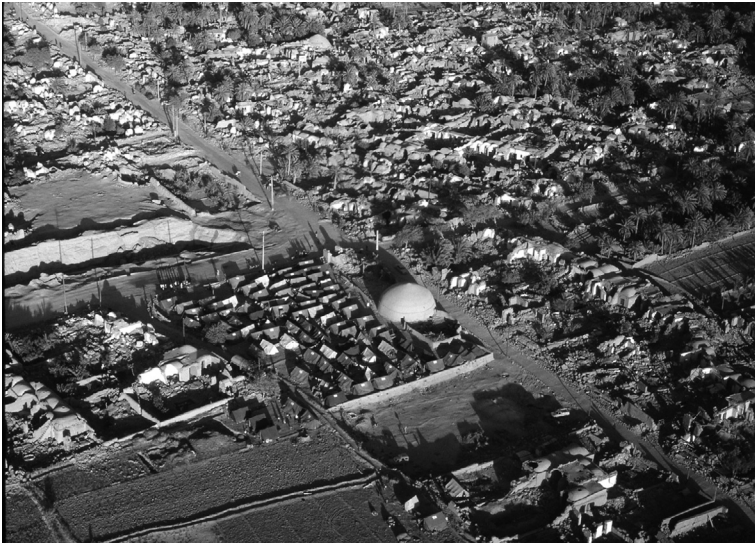
PLATE 13.11 Destruction of the Tabas-e Golshan oasis town by the 16 September 1978 M_w 7.3 earthquake. Only a few domed structures withstood the earthquake. See Figure 13.8 for the location. Photographed on 28 September 1978.
