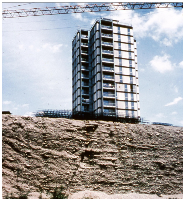
PLATE 1 Apartment building built on a recent fault through Quaternary alluvial deposits in northern central Tehran. Photographed in 1983.
