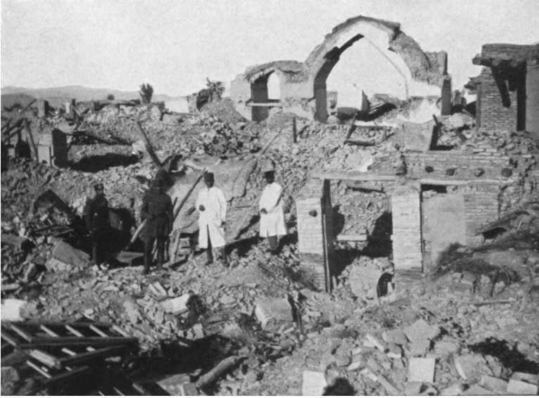
PLATE 12.3 The 1930 ruined mosque at Dilmān (Salāms). Only sections of the portal arches and thick load-bearing masonry pillars are standing. For the location, see Figure 12.5 . Courtesy Yahyā Zokāʾ from an unknown photographer.
