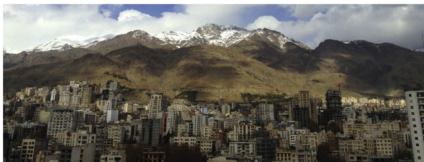
PLATE 2 Buildings in northern Tehran constructed on the active North Tehran Thrust, as well as on the hanging-wall block of the thrust fault. Photographed in 2013 (Courtesy of R.Q.M. Tābān).
