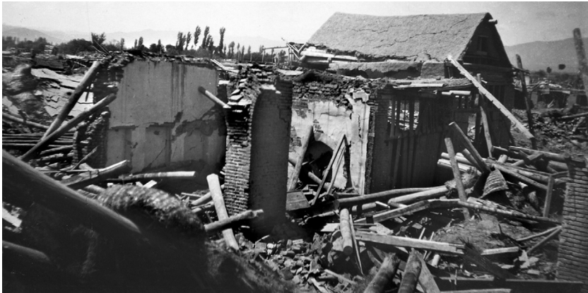
PLATE 12.2 Historic photograph of the 1930 destruction at Dilmān (Salāms) showing the type of structures. Only the load-bearing masonry pillars and thick walls are standing. Wooden beams of the collapsed ceilings are scattered in the debris. For the location, see Figure 12.5 . Courtesy Yahyā Zokā' from an unknown photographer.
