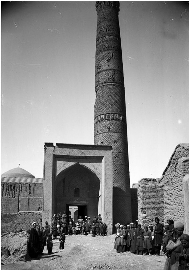
PLATE 13.17 The minaret of the congregational mosque (Menāreh-ye Kabir) at the town of Tabas-e Golshan photographed in 1906 by Sven Anders Hedin (Hedin, 1910; see Figure 13.8 for the location). The minaret, which was possibly built in 993–1014 (late Ghaznavid-early Saljuq), collapsed on 22 February 1907 due to construction of the Kariz-e Allāhābād (qanāt), which weakened the foundation of the minaret (Meshkati, 1970; Daneshdoust, 1998). The survival of the minaret for a period of >900 years indicates the lack of large-magnitude earthquakes since at least the year 1000. Courtesy of the Sven Hedin Foundation, Stockholm, Sweden, published with permission.
