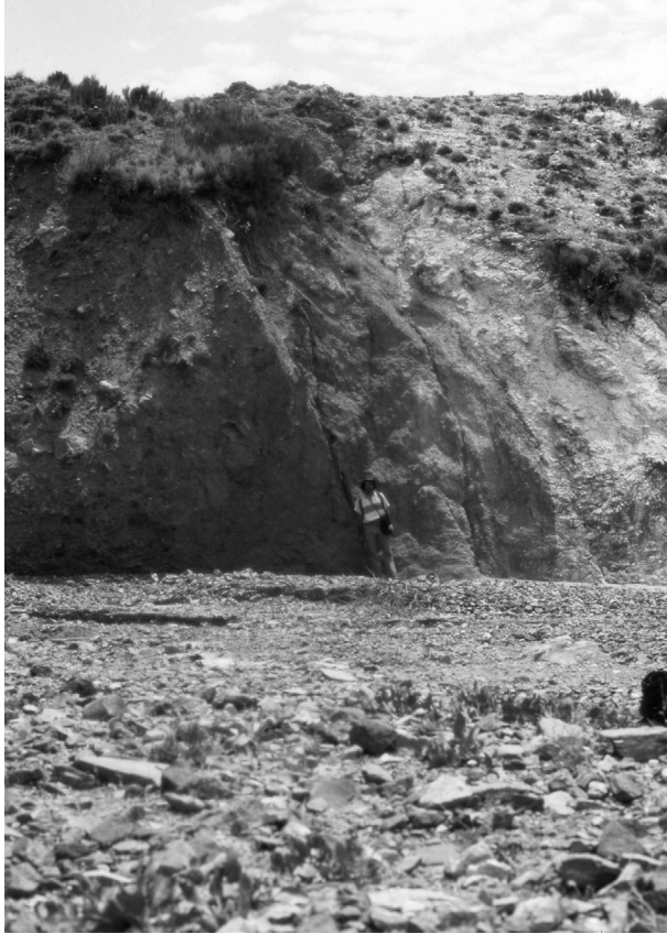
PLATE 11.9 Recent faulting along the Germirud River. The west southwestern block of Miocene rocks (right) is thrust over the east northeastern Quaternary alluvial deposits (left). Photographed in 1975. For location, see Figure 11.14 .
