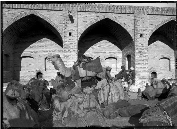
PLATE 13.20 The Robāt-e Gur caravanserai built with thick load-bearing abutments supporting the lateral thrust constructed sometime during the Qājār period (1779–1925). The structure was located about 43 km northwest of Tabas-e Golshan and 47 km to the northwest of the 1978 coseismic surface faulting, and was destroyed during the earthquake. Photographed in 1906 by Sven Hedin. Published with permission from the Sven Hedin Foundation, Stockholm, Sweden; http://svenhedinfoundation.org .
