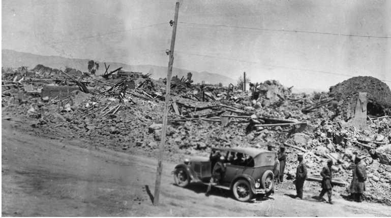
PLATE 12.1 Historic photograph of the 1930 earthquake ruined city of Dilmān (Salāms; rebuilt as Shāpur). The buildings were adobe and brick structures with wooden beams used in the roof. Courtesy Yahyā Zokā' from an unknown photographer.
