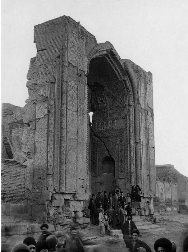
PLATE 11.6 Outer portal of the Tabriz Blue mosque (masjed-e Kabud/Jahānshāh; built in 1465) severely damaged by the 1780 earthquake. Note the massive adobe brick walls, clad with kiln tiles, disintegrated by the strong ground shaking of the 1780 Tabriz earthquake. Note the deep fractures developed in very thick walls of this splendid fifteenth-century structure. The well-constructed portal did not collapse, whereas the modern buildings in Iran have been leveled to the ground during recent earthquakes. Photographed in 1906 by Sven Hedin (published with permission from the Sven Hedin Foundation, Stockholm, http://svenhedinfoundation.org ).
