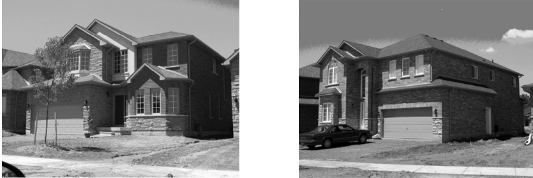
Figure 5-11 Applications of masonry and stone veneer.
