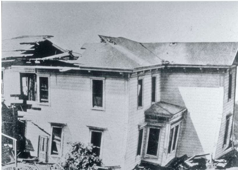
Figure 1-6 A house damaged due to fault movement. The fault passed under this house near Wright's Station, on the Southern Pacific Railroad, in Santa Cruz County, California. The house was severed by fault movement during the earthquake. Photo credit: R.L. Humphrey, U.S. Geological Survey.
