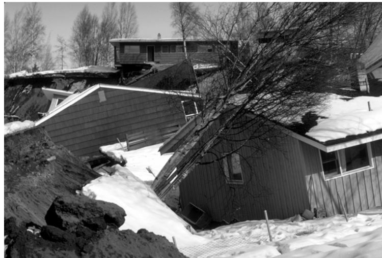
Figure 1-7 Houses damaged due to a landslide at the site. Photo Courtesy National Information Service for Earthquake Engineering, University of California, Berkeley
