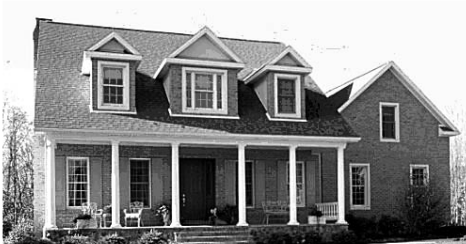
Figure 5-14 House constructed with masonry walls.
