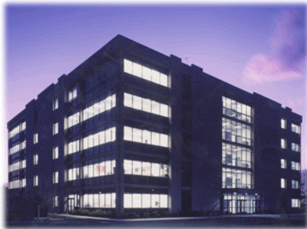
Figure 5-7 Sample new school building design in Salt Lake City K-12 School District.
