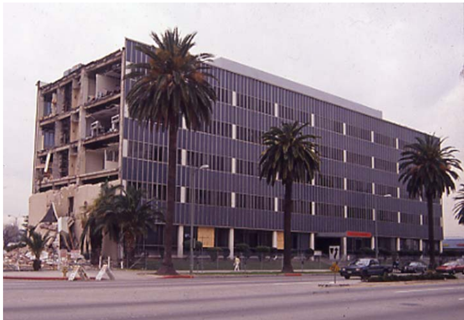
Figure 6-3 Partially collapsed end-wall in 5-story office building caused by severe earthquake ground shaking. (C. Arnold photo)
