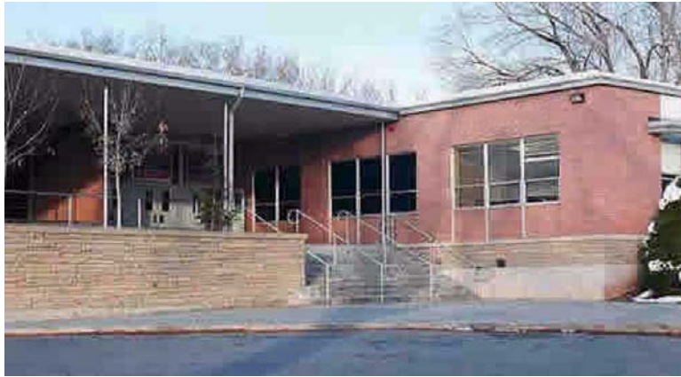
Figure 5-6 Sample existing school building in Salt Lake City K-12 School District.
