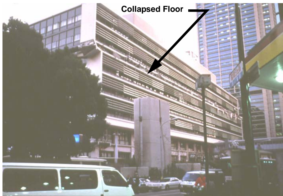
Figure 3-2 Eight-story reinforced-concrete-frame office building in Kobe, Japan that partially collapsed during the magnitude-7.8 earthquake of January 17, 1995. Note that the sixth floor is missing, due to collapsed columns at that level. Seismic codes in Japan are essentially equivalent to those in the United States. (photo courtesy of C. Rojahn)
