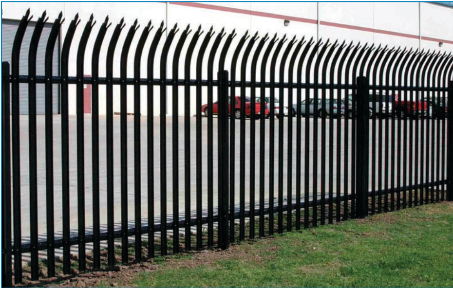
Figure 4-32: Crash-rated fence.
