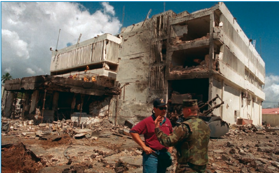
Figure 1-17: Damage to the U.S Embassy, Tanzania
