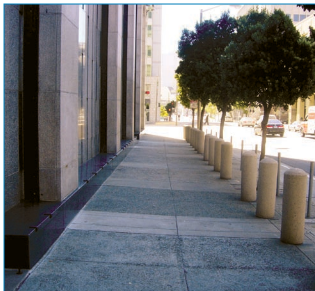
Figure 6-8: A well-designed zero-setback protection. The engineered bollards define the transition between the first and second layers of defense and the street trees soften the intrusion of bollards.
