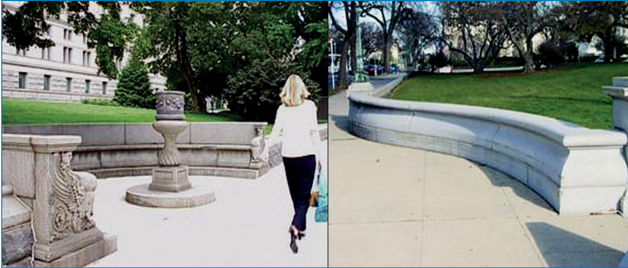
Figure 6-14: Barriers in harmony with the architecture. The seating (left) and the serpentine wall (right) are engineered barriers.
