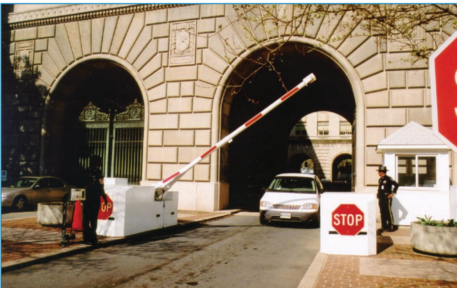
Figure 4-42: Drop-arm crash beam.
