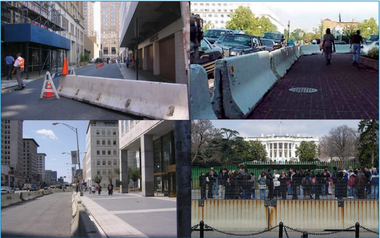
Figure 1-4: Jersey barriers installed in New York City and Washington D.C. after 9/11.
