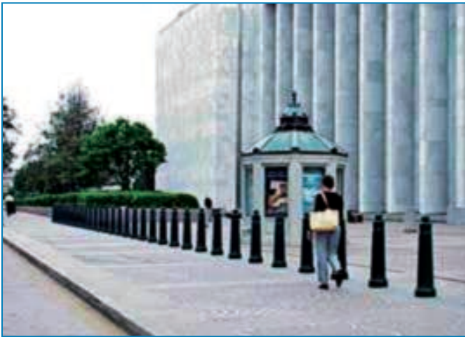
Figure 4-4: These bollards resemble a wall. SOURCE: NCPC)
