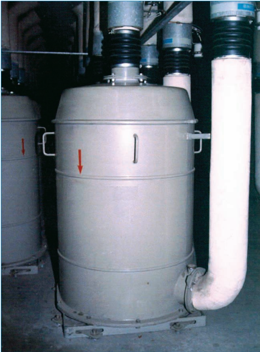
Figure 3-4 A canister-type filter unit is often used for Class 1 Safe Rooms to maximize storage life of the filters.
