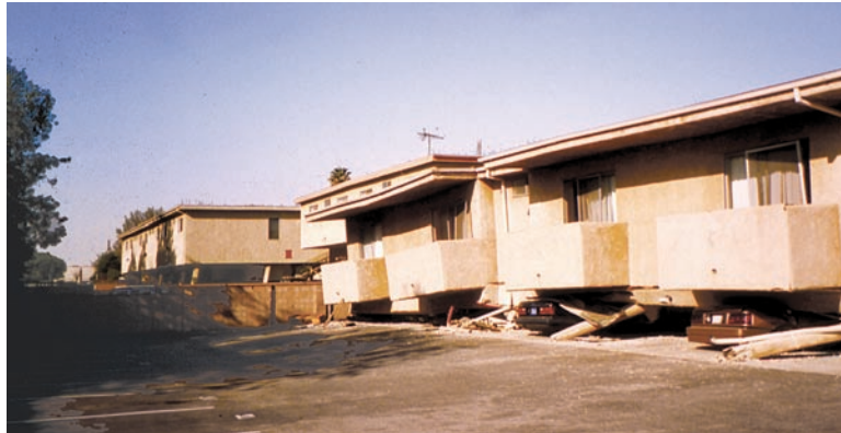
Figure 8-4: A 1970s building type with a deficiency not prohibited by the code at the time—a tuck-under apartment with parking at the ground level, creating a weak story. Many of these buildings collapsed in the Northridge earthquake. Sixteen deaths occurred in the Northridge Meadows apartments, or 42% of those directly killed by the earthquake.
