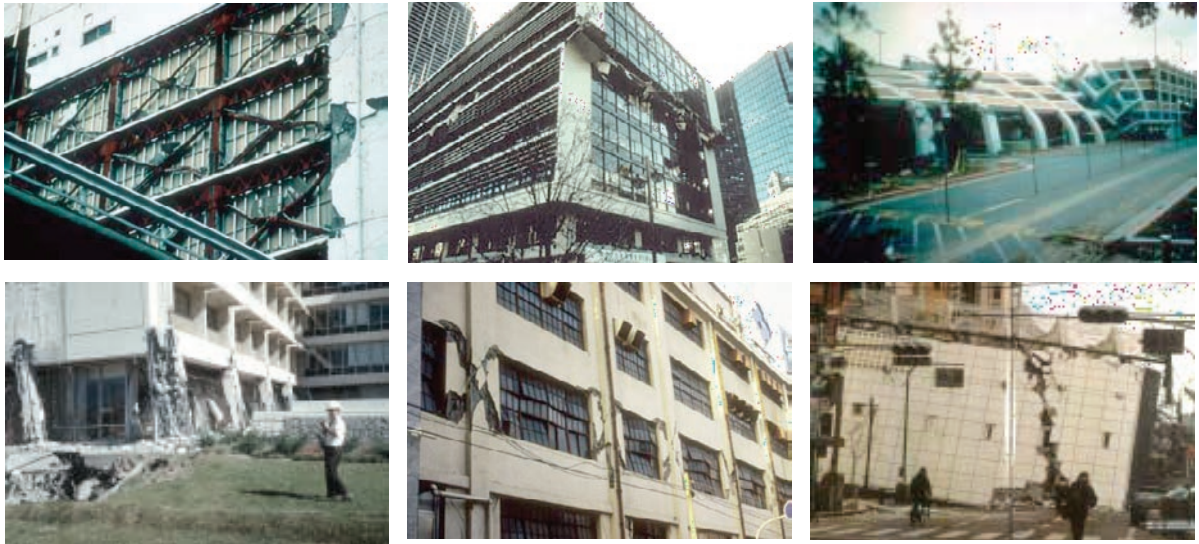
Figure 7-12: Examples of typical earthquake damage.
