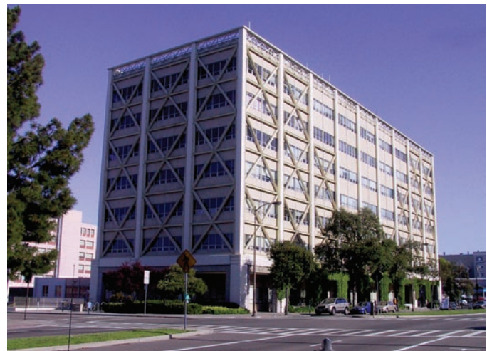
Figure 8-15: Renovation and retrofit of a concrete warehouse structure by removing the exterior wall, inserting steel braces and window wall, and adding several floors.
