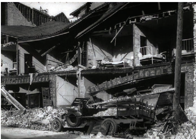
Figure 6-2: Santa Barbara, 1925, typical failure of brick walls and timber interior.
