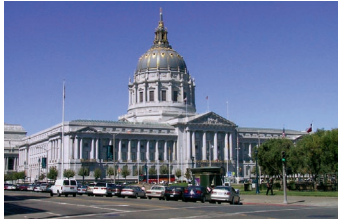
Upper left: Oakland City Hall (Engineer: Forell/Elsesser). Upper right: San Francisco City Hall (Engineer: Forell/Elsesser). Bottom: Hearst Mining Building at University of California, Berkeley (Engineer: Rutherford & Chekene). Installation of an isolation system under an existing building is complex and often expensive, but the system minimizes the need to disrupt historic fabric in the superstructure with shear walls or braces, and is designed to protect the superstructure from significant damage in a major event.
