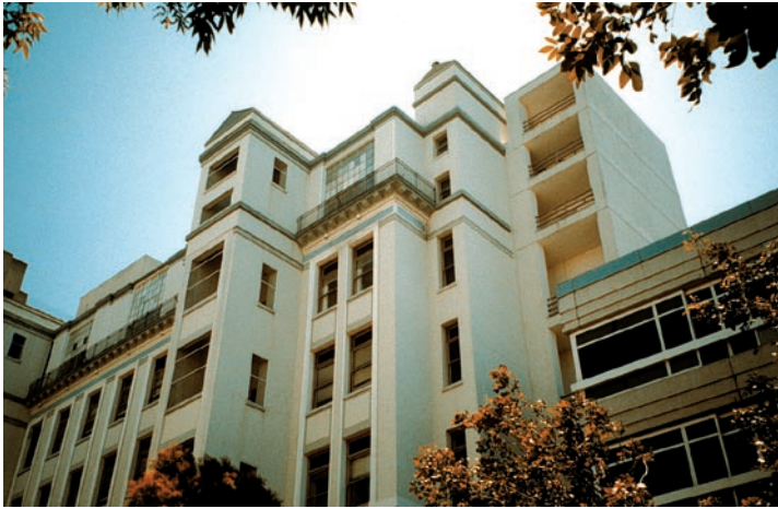
Figure 8-12: External towers were added to strengthen this building from the outside. The new tower is the element at center-left of the figure. The retrofit scheme for this building is discussed in detail in Figure 8-9.
