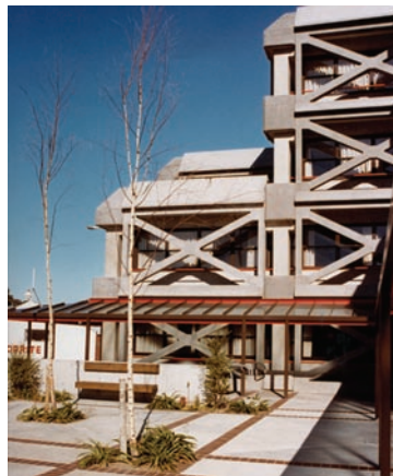
Figure 5-42: Exposed cross-bracing examples.
