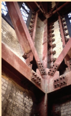
Figure C: Steel space frame inserted within tower
