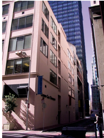
Figure 8-18: Infill of certain panels of an exterior wall for strengthening. Originally on the alley wall, only the central stair tower was solid wall, and elsewhere the upper window panel pattern was typical to the street.
