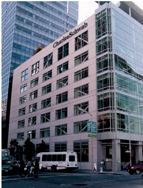
Figure 8-15: Renovation and retrofit of a concrete warehouse structure by removing the exterior wall, inserting steel braces and window wall, and adding several floors.
