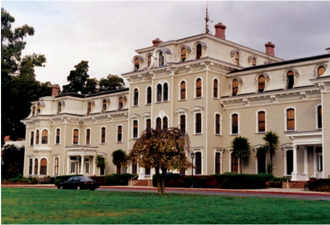
Figure 8-21: Mills Hall, Mills College, California. Structure is wood studs and sheathing. Interior shear walls were created by installing plywood on selected interior surfaces.
