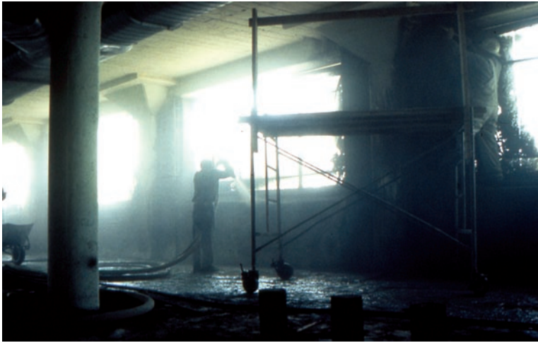
Figure 8-10: Intense construction activity and disruption from interior shotcrete.
