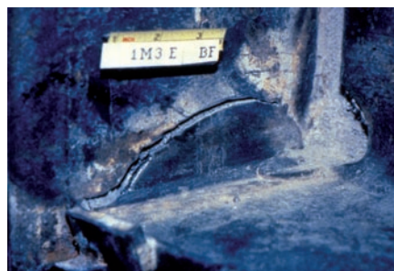
Figure 8-3: An example of a recently designed building with seismic deficiencies not understood at the time of design. In this case, the deficiency was “pre-Northridge” moment-frame connections, which proved to be extremely brittle and unsatisfactory. Hundreds, if not thousands, of these buildings were designed and built in the two decades before the Northridge earthquake (1994).
