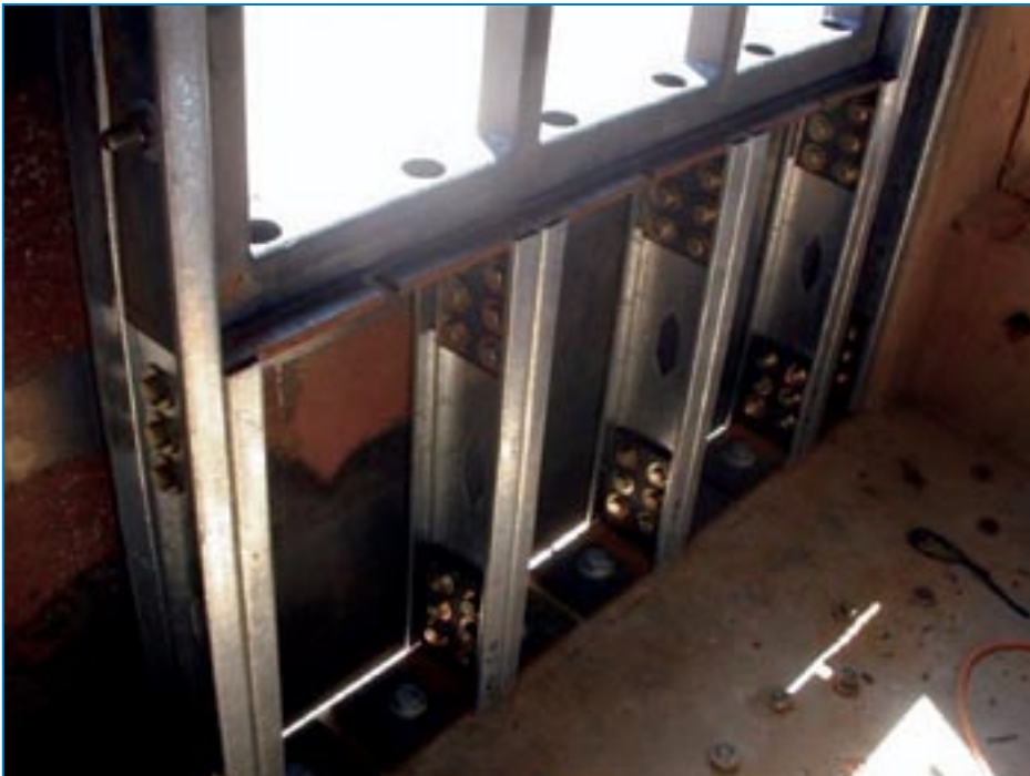
Figure 3-12: Metal stud blast wall.
