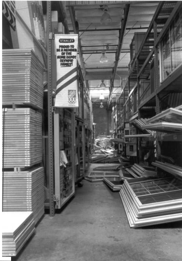
Figure 2-4 Contents spillage in the door/window area of a Santa Clarita store.
