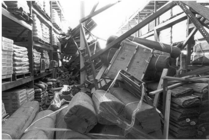
Figure 2-1 Cross-aisle collapse in the building materials section of the Santa Clarita store.
