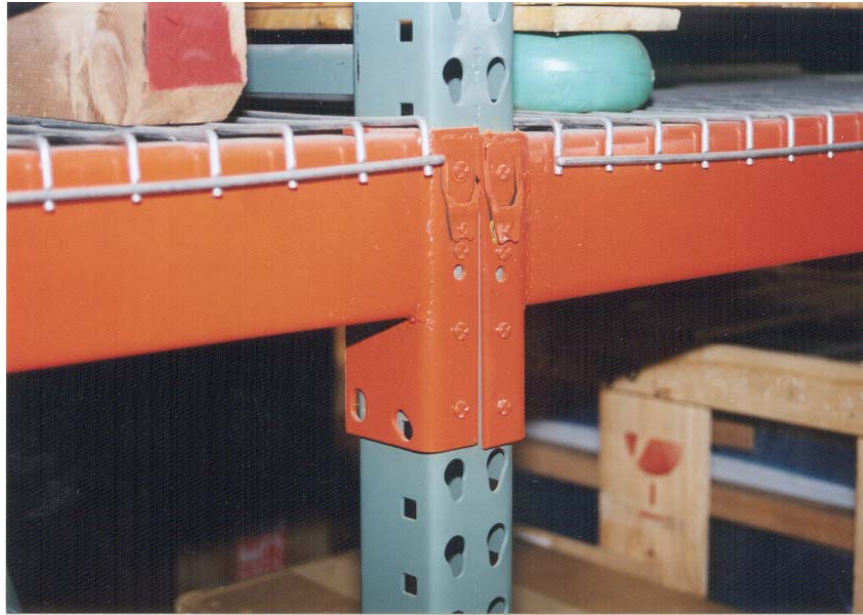
Figure 1-3 Typical proprietary moment connection.
