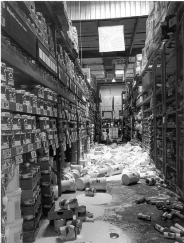
Figure 2-6 Contents spillage in the paint area of a Santa Clarita store.
