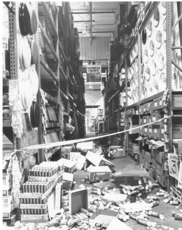
Figure 2-7 Contents spillage in a small-items section of a Santa Clarita store.
