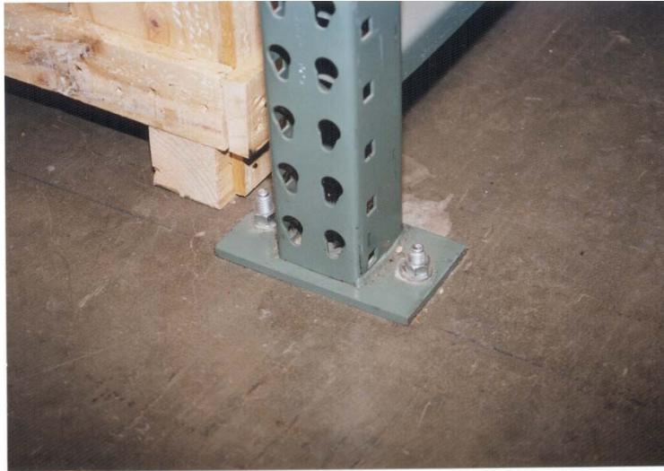
Figure 1-5 Typical column base plate connection.
