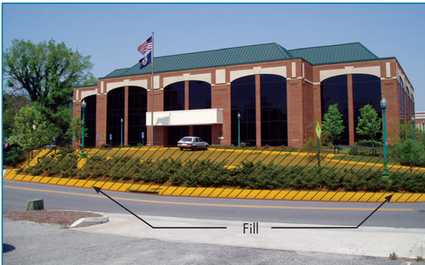
Figure 2-24: Municipal building elevated on fill
