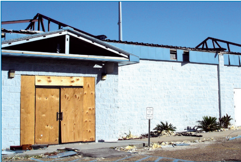
Figure 4-41: Longbeach Police Station
