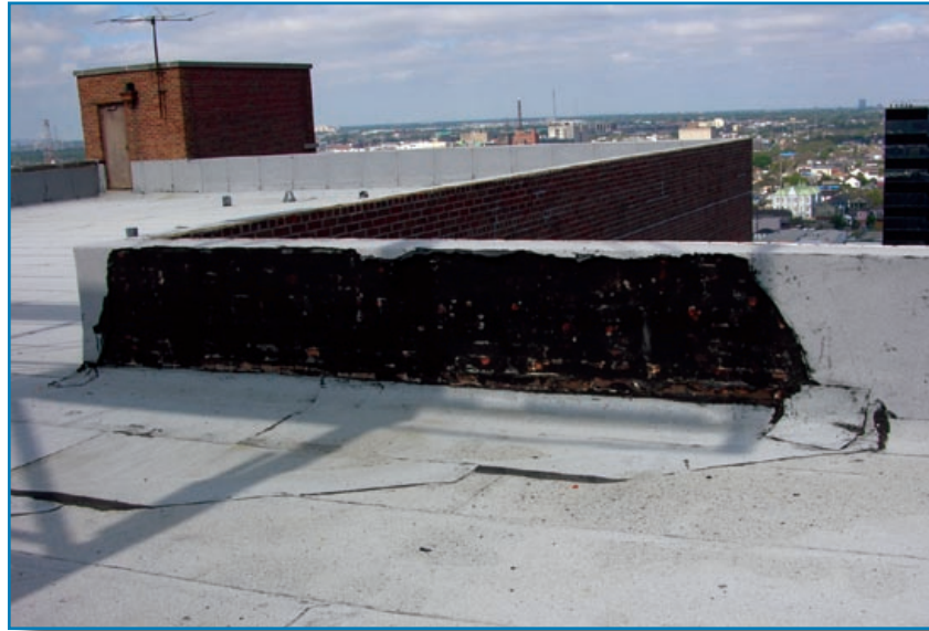
Figure 3-117: Failed base flashing adhered directly to the brick parapet. Hurricane Katrina (Louisiana, 2005)
