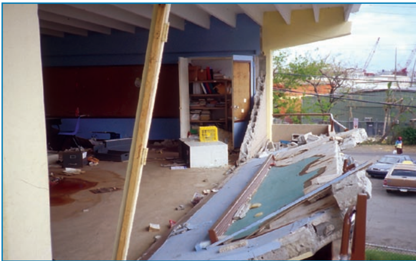
Figure 3-15: The unreinforced CMU wall collapsed at a school during Hurricane Marilyn. (U.S. Virgin Islands, 1995)
