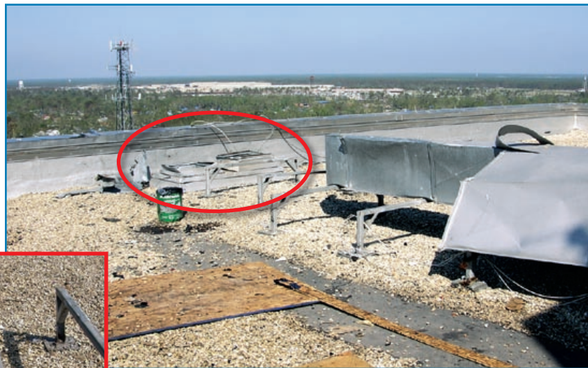
Figure 3-72: Two large openings remained (circled area and inset to the left) after the ductwork on this roof blew away. Hurricane Katrina (Mississippi, 2005)
