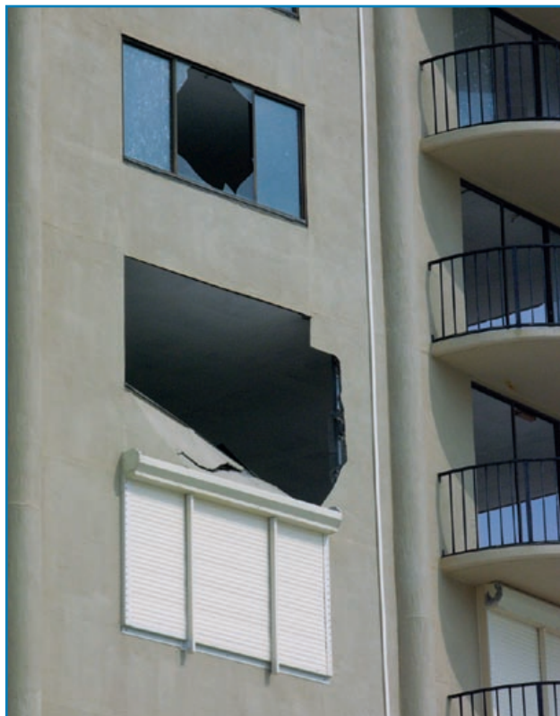
Figure 3-113: The lower window assembly was protected with a motorized shutter. Hurricane Ivan (Florida, 2004)
