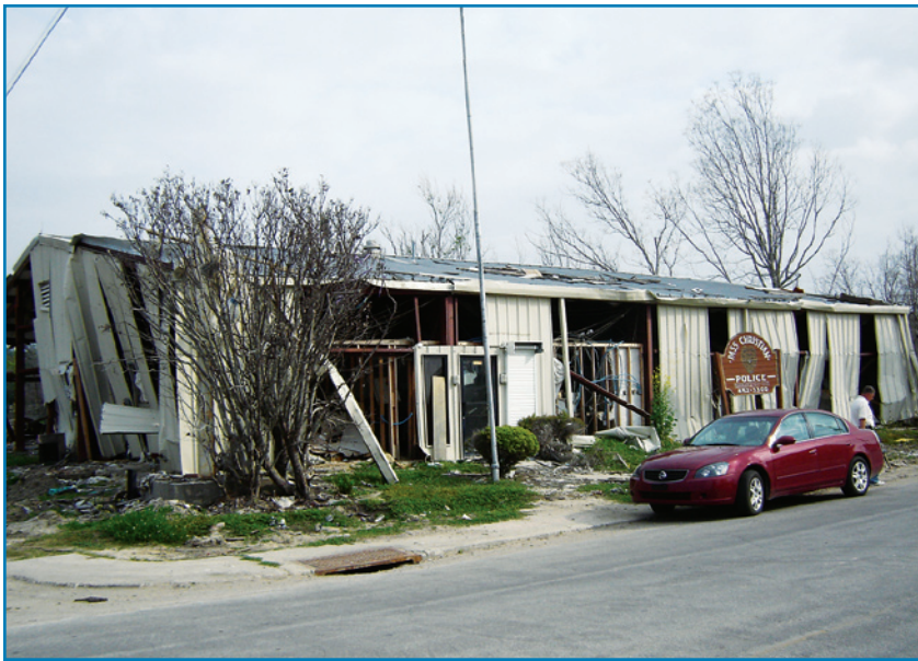
Figure 4-32: Police station in Pass Christian
