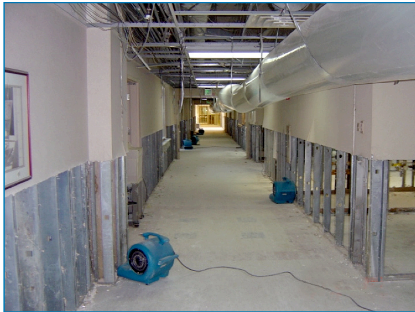
Figure 4-15: Drying of flooded ground floor at Hancock Medical Center
