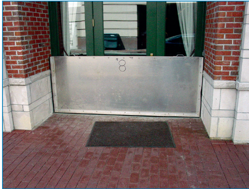
Figure 2-36: Example of an aluminum flood barrier used for flooding less than 3 feet deep.
