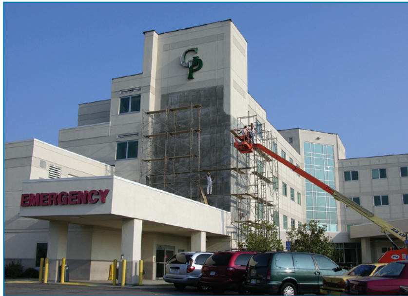
Figure 4-6: Repair of EIFS wall covering on Garden Park Medical Center
