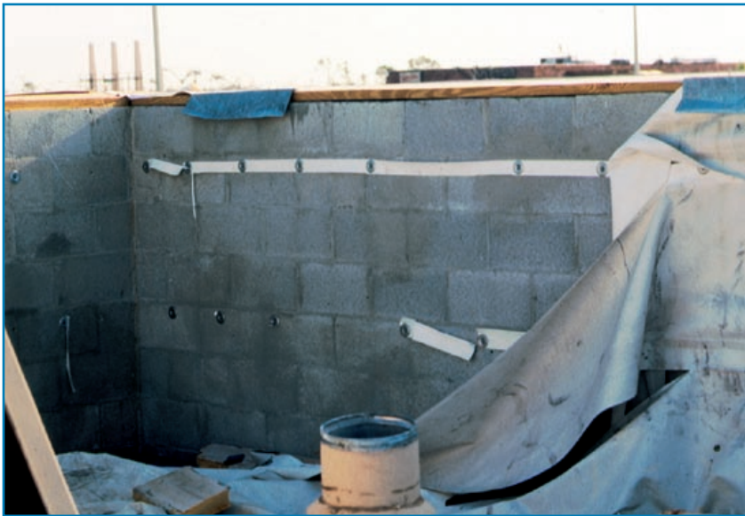
Figure 3-66: If mechanically attached base flashings have an insufficient number of fasteners, the base flashing can be blown away. Hurricane Andrew (Florida, 1992)
