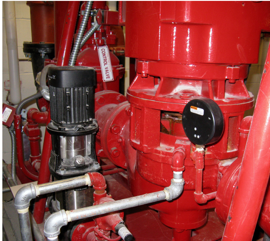
Figure 4-3 A typical jockey pump.
