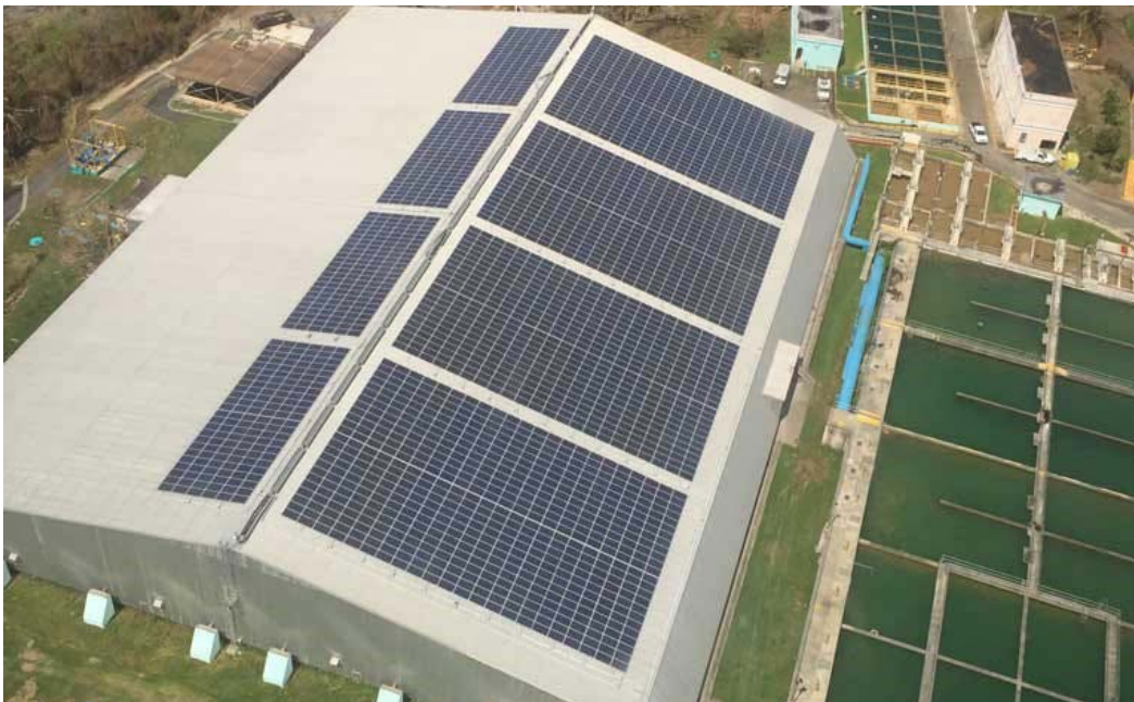
Figure 4.2.5. Installing renewable energy resources like solar panels can provide a standby source of power for wastewater treatment facilities. (National Renewable Energy Laboratory [NREL], 2017)
