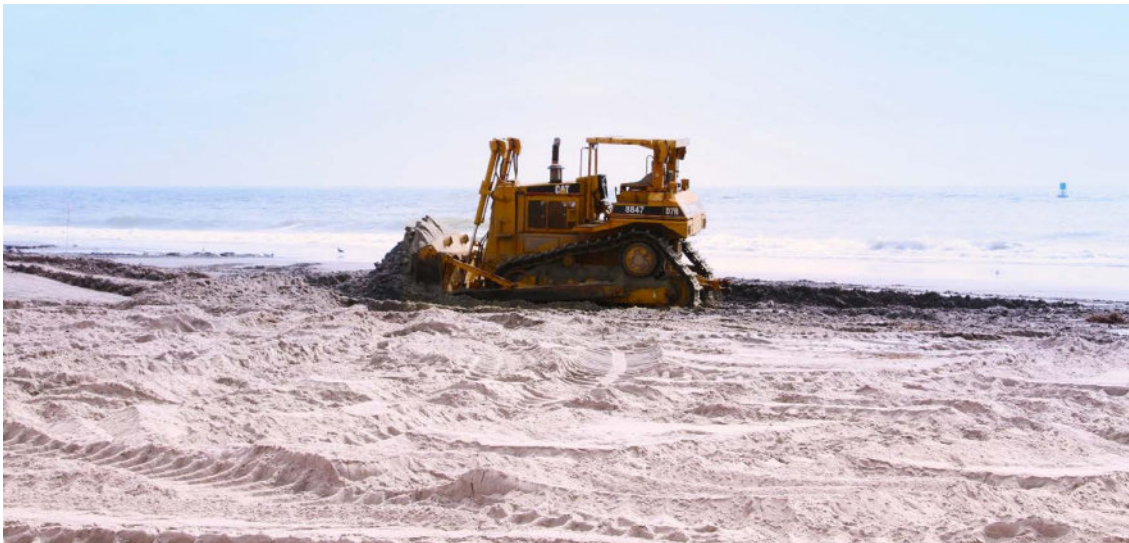
Figure 5.4.7. Beach nourishment replaces sand lost through longshore drift or erosion and increases resilience. (Source: USACE, 2020).
