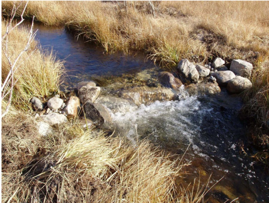
Figure 2.1.4. Energy dissipators such as stone drop structures can help slow the movement of water to decrease erosion and scour. (NRCS, No Date)
