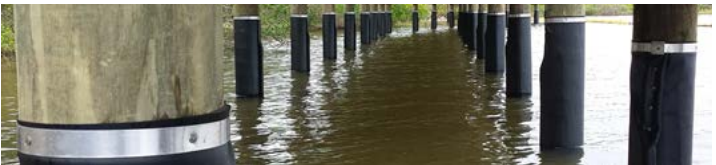
Figure 5.5.1. Piles can be wrapped with PVC to protect them from damage (Source: Marine Fix Supply, 2018).
