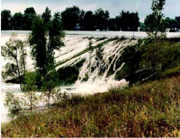
Figure 2.3.10. Initial embankment overtopping can lead to a complete overflow. (Source: USFWS, 2008)
