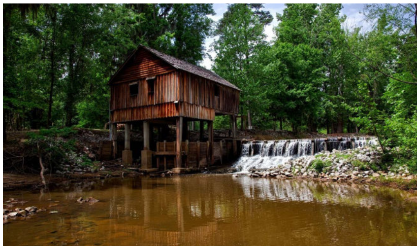
Figure 2.3.1. This dam is considered low hazard potential because, if it failed, it would only impact the forest around it. (Source: Library of Congress, Prints & Photographs Division, photograph by Carol M. Highsmith, LC-DIG-highsm-08052)
