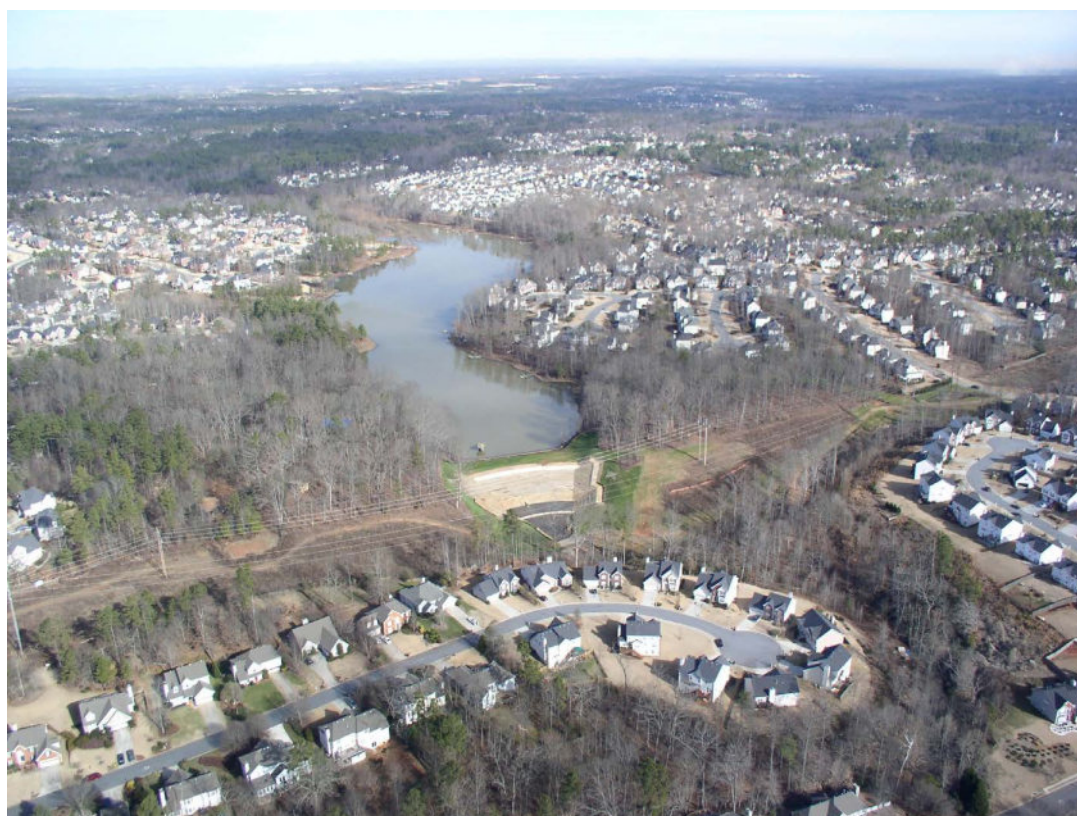
Figure 2.3.2. This dam is considered high hazard potential because its failure would impact the community directly downstream and could result in loss of life and property. (Source: NRCS, 2014)
