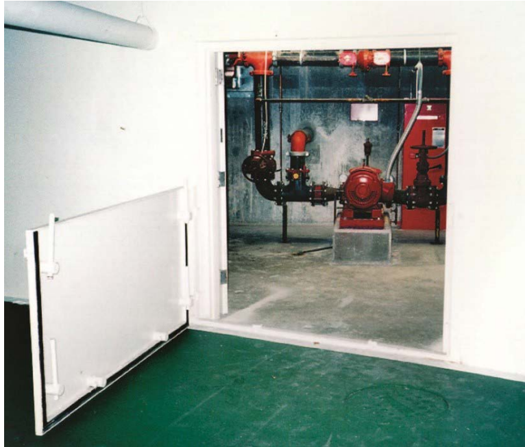
Figure 4.1.4. Water-tight doors can be used to protect pumps and other equipment in pump houses and booster stations.
