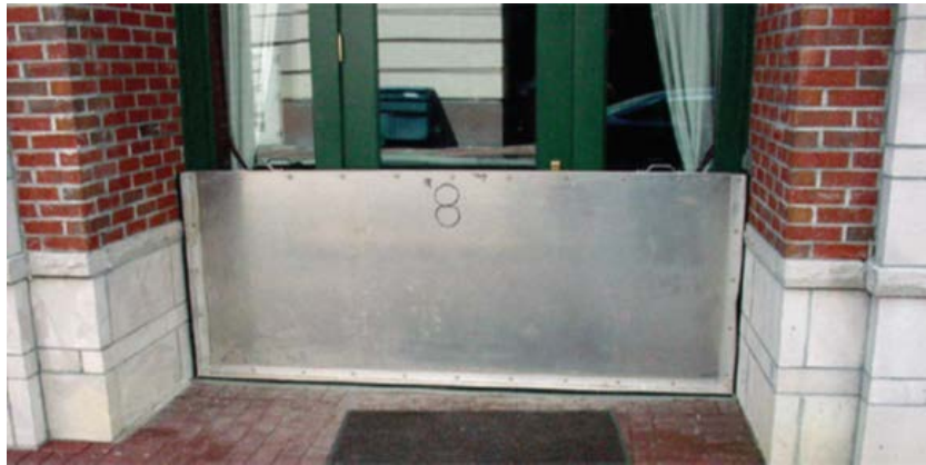
Figure 5.2.4. Flood gates and flood barriers can help protect buildings and structures against rising water.
