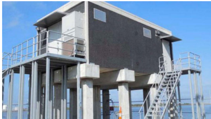
Figure 4.3.9. Elevating a control house in coastal areas can protect it against damage from storm surge and flooding. (Source: Modular Connections, 2020)
