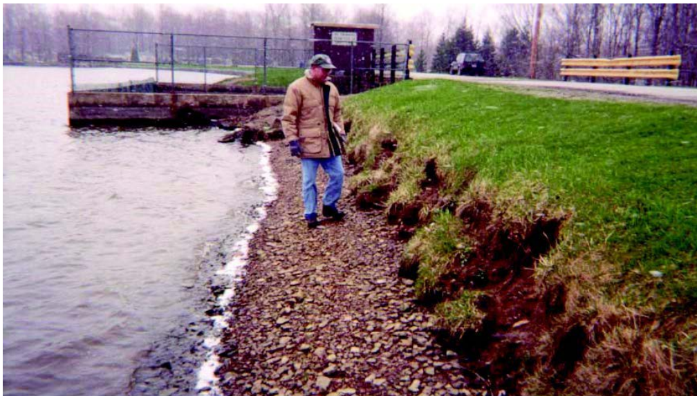
Figure 2.3.9. Wave action can erode the upstream slope of a dam. (Source: USFWS, 2008)
