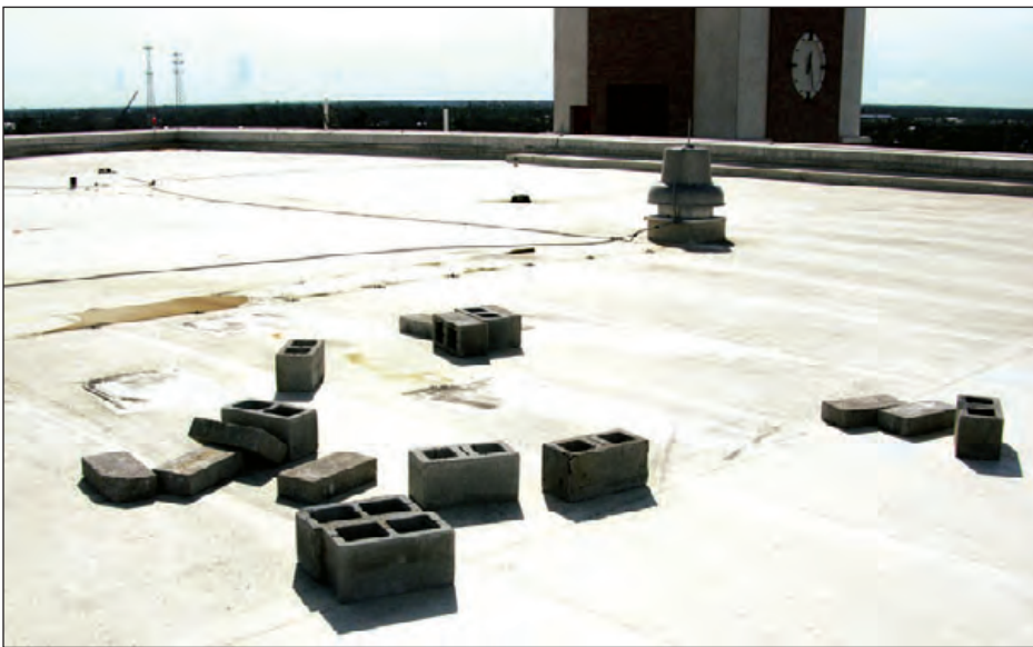
Figure 6-108: A satellite dish anchored similarly to that shown in Figure 6-107 was blown off this five-story building. Estimated wind speed: 140–160 mph. Hurricane Charley (Florida, 2004)
