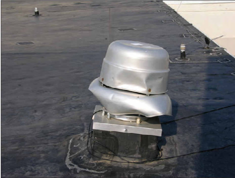
Figure 6-103: This exhaust fan was impacted by wind-borne debris. Although it is often impractical to place all equipment such as fans in penthouses, doing so to the extent possible avoids debris damage. Estimated wind speed: 130 mph. Hurricane Katrina (Mississippi, 2005)
