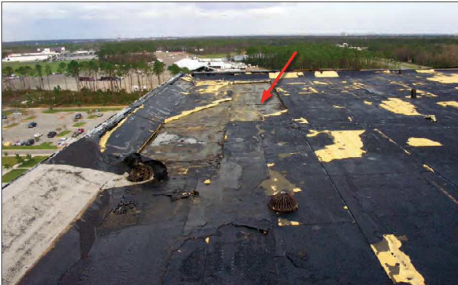
Figure 6-68: The blown off insulation (red arrow) may have initiated blow-off of the roof membrane. Estimated wind speed: 105–115 mph. Hurricane Ivan (Florida, 2004)
