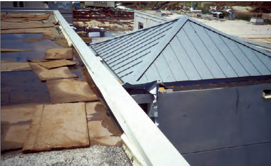
Figure 6-9: The irregularity created by the stair tower (covered with a metal roof) caused turbulence resulting in wind speed-up and roof damage. Hurricane Andrew (Florida, 1992)
