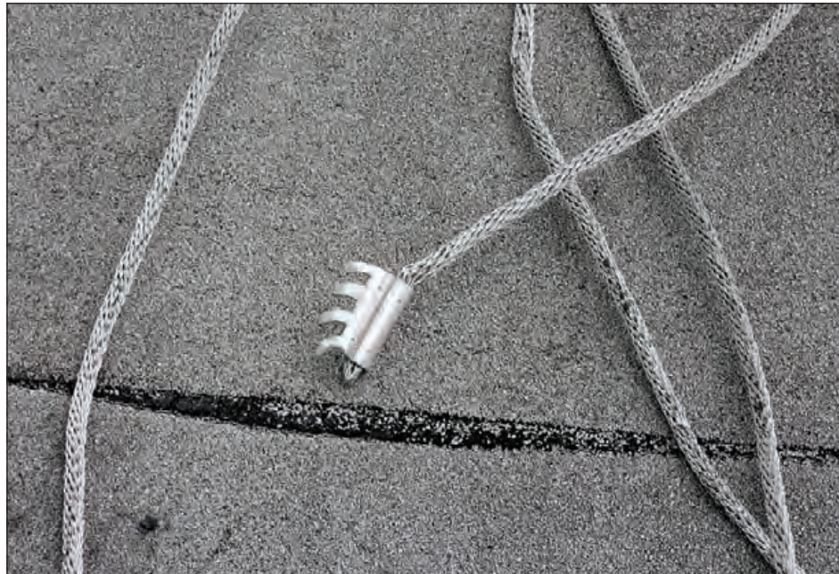
Figure 6-116: If conductors detach from the roof, they are likely to pull out from pronged splice connectors. Estimated wind speed: 90–100 mph. Hurricane Charley (Florida, 2004)
