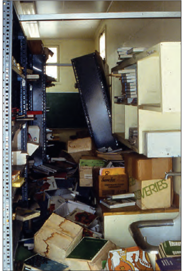
Figure 4-8: Fallen filing cabinets and shelves, Northridge, CA, 1994
