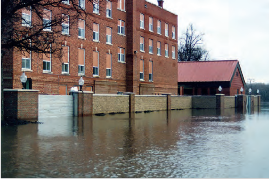
Figure 5-29: A masonry floodwall with multiple engineered openings in Fargo, ND, during flooding in 2001
