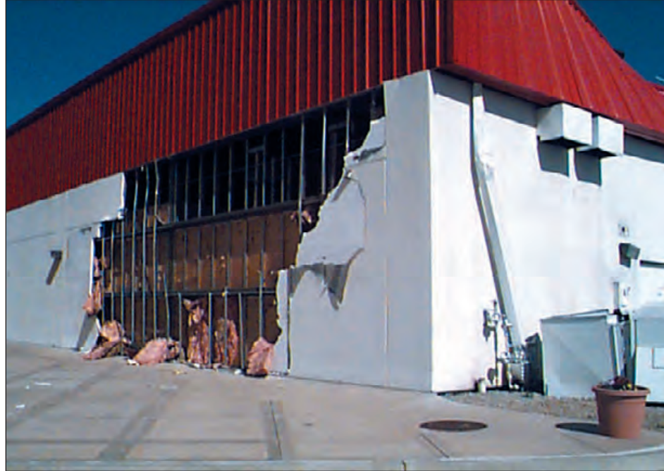
Figure 6-61: EIFS blow-off near a wall corner. At one area, the metal fascia was also blown in.
