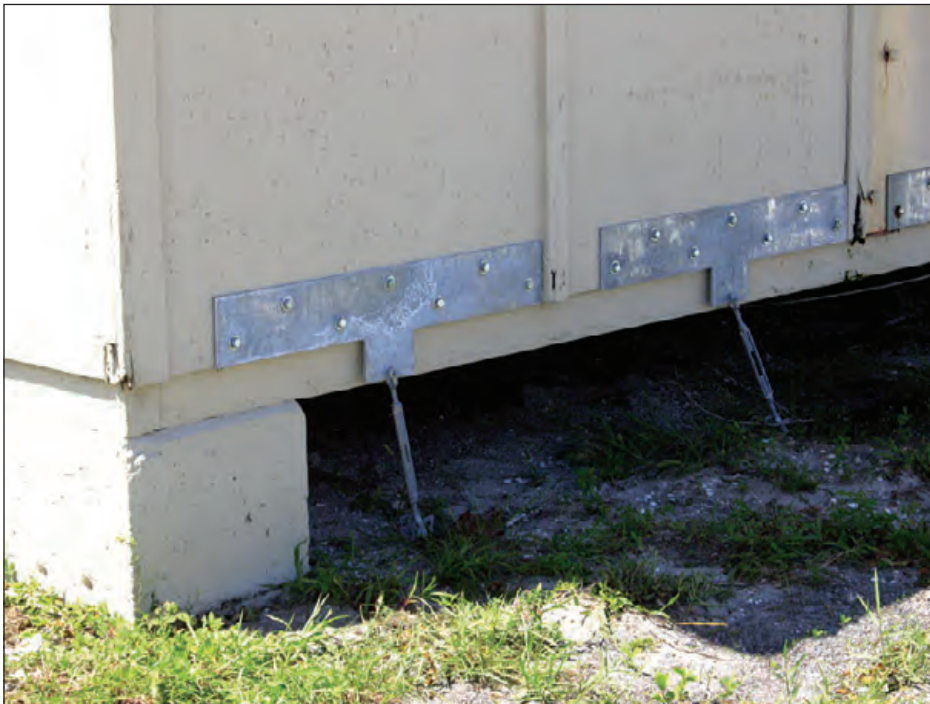
Figure 6-27: Unlike the portable classroom shown in Figure 6-22, with the thick T-shaped plates and taut turnbuckles, this portable classroom has a robust anchorage to the ground. Hurricane Francis (Florida, 2004)
