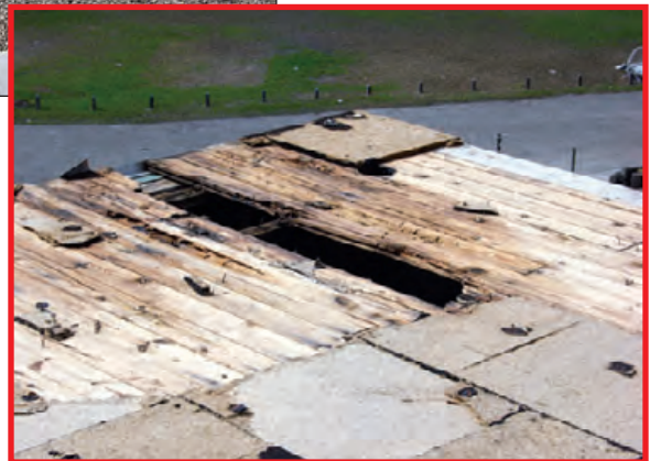
Figure 6-131: The built-up roof on this school was blown off after a few of the rotted wood planks detached from the joists. Estimated wind speed: 120 mph. Hurricane Katrina (Mississippi, 2005)
