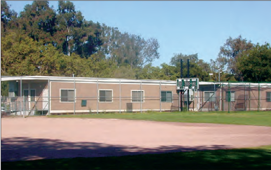
Figure 1-8: Typical portable classrooms, 1980s, still in use
