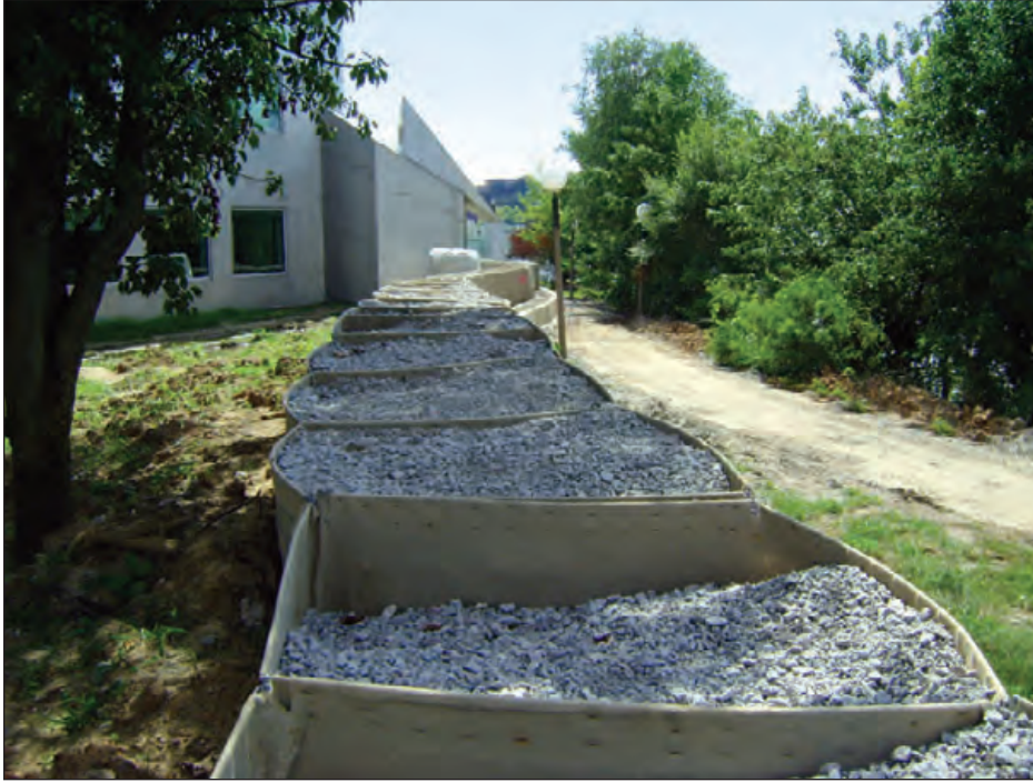
Figure 5-31: Gravel-filled containers form a barrier to protect the University of Iowa (2008)
