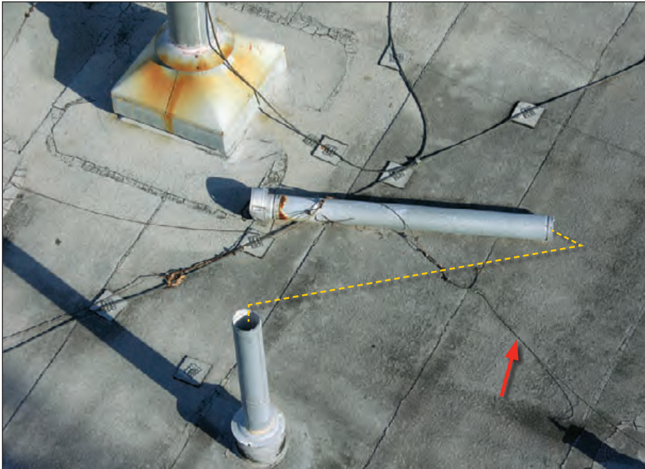
Figure 6-97: Guyed flue blew over (red arrow indicates one of the guys). Estimated wind speed: 92 mph. Hurricane Ike (Texas, 2008)
