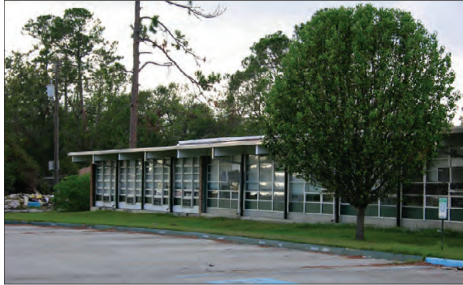
Figure 6-124: On-site water-spray testing in accordance with ASTM E 1105 can be used to evaluate wind-driven rain resistance. Older window assemblies such as the ones at this school are often quite susceptible to leakage. Estimated wind speed: 125 mph. Hurricane Katrina (Mississippi, 2005)
