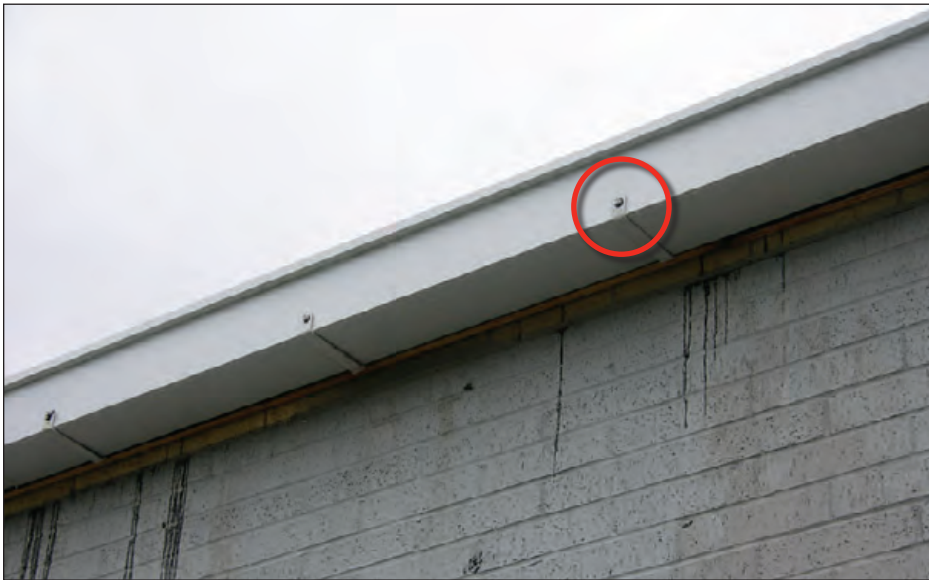
Figure 6-76: At this gutter, a fastener connected the bracket to the gutter. Note: To avoid leakage at the fasteners between the bracket and gutter, the bracket should extend near or to the top of the gutter so that the fastener would be above the waterline. Estimated wind speed: 95 mph. Hurricane Ike (Texas, 2008)
