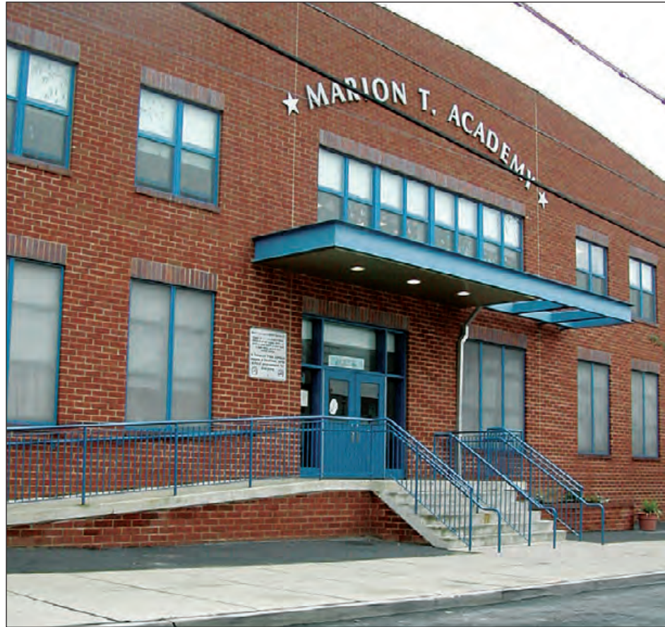
Figure 5-23: A stemwall foundation elevates the Marion T. Academy above the flood level in Wilmington, DE.
