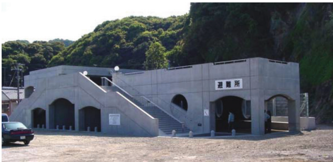
Figure A-7 Tsunami refuge in Kaifu, Japan.
