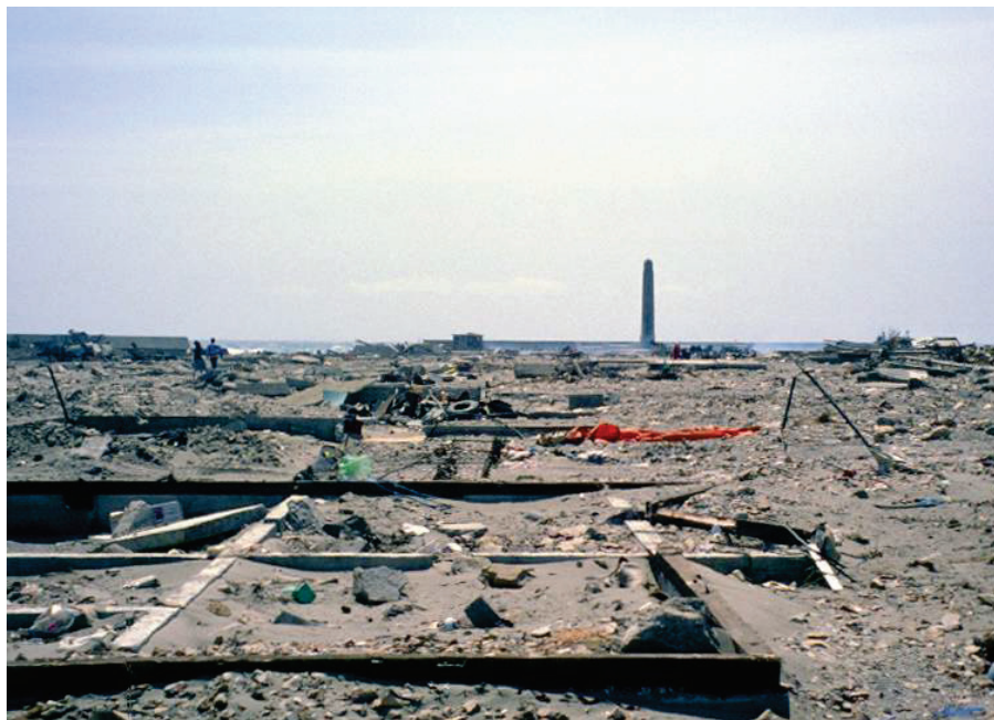
Figure 2-10 Total destruction of a group of wood-frame houses in Aonae Village, Okushiri Island, Japan, 1993 Okushiri tsunami (photo courtesy of H. Yeh).
