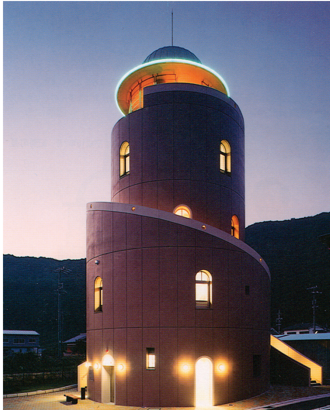
Figure A-5 Nishiki Tower in Kise, Japan.
