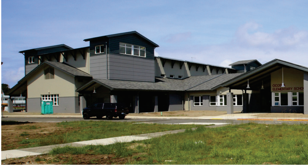
Figure 3-5 Tsunami evacuation refuge over a cafeteria and gymnasium at Ocosta Elementary School, Westport, Washington (photo courtesy of P. Akerlund).
