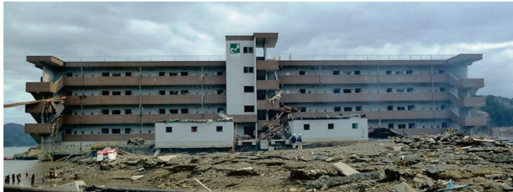
Figure 6-2 Reinforced concrete apartment building designated as a vertical evacuation structure in Minamisanriku, Japan, 2011 Tohoku tsunami.
