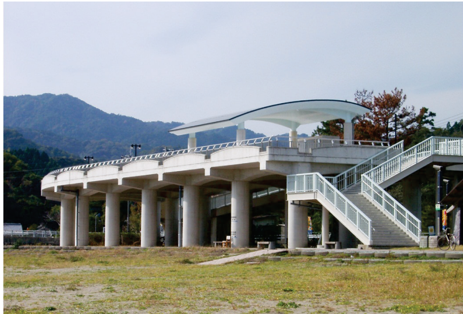
Figure A-6 Refuge at Shirahama Beach Resort, Japan (photo courtesy of N. Shuto).
