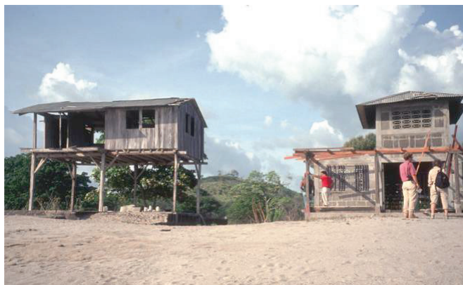
Figure 2-11 Beach houses with varying levels of damage in El Popoyo, Nicaragua, 1992 Nicaragua tsunami (photos courtesy of H. Yeh).
