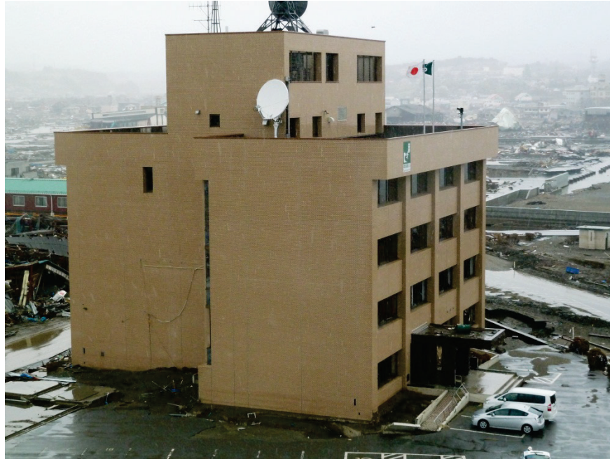
Figure A-4 Successful designated vertical evacuation building in Kesennuma Port, Japan.
