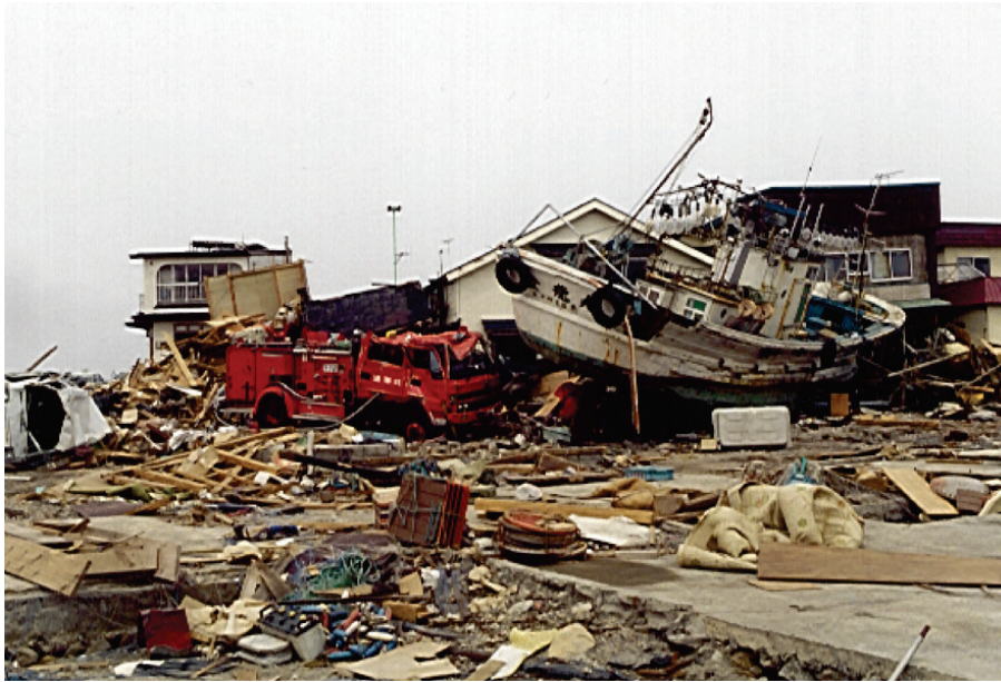
Figure 2-12 Damage caused by impact from water-borne debris (fishing boat) in Aonae, Japan, 1993 Okushiri tsunami (photo courtesy of J. Preuss).
