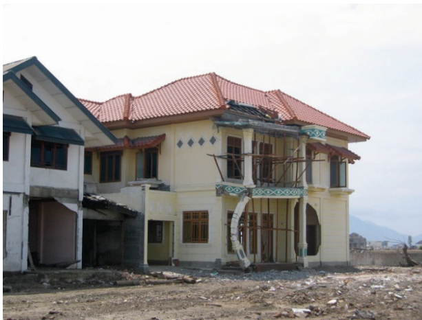
Figure 2-17 Damage to non-engineered concrete columns due to debris impact, 2004 Indian Ocean tsunami (photos courtesy of M. Saatcioglu, A. Ghobarah, and I. Nistor, CAEE, 2005).
