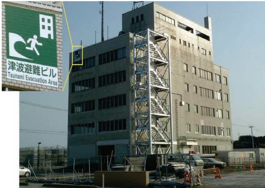
Figure 9-1 Five-story building in Kesenuma, Japan, with an exterior metal staircase installed to provide unobstructed access to the refuge area on the roof (Fraser et al., 2012).
