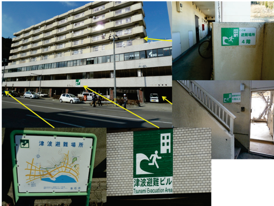
Figure 4-5 Residential apartment building in Kamaishi, Japan, with a designated refuge area at or above the fourth level.
