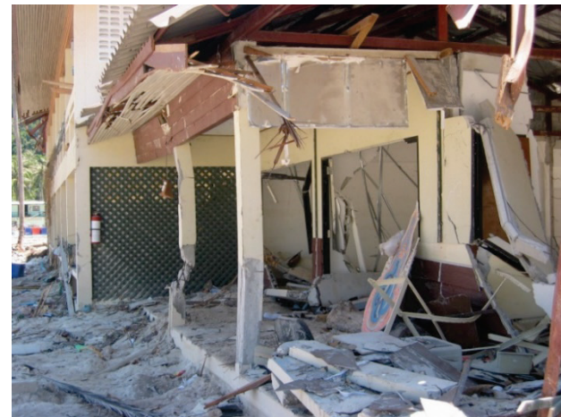
Figure 2-17 Damage to non-engineered concrete columns due to debris impact, 2004 Indian Ocean tsunami (photos courtesy of M. Saatcioglu, A. Ghobarah, and I. Nistor, CAEE, 2005).
