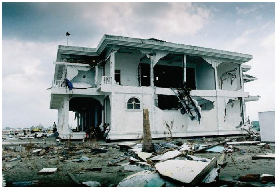
Figure 2-15 Example of surviving reinforced concrete mosque in Uleele, Banda Aceh, Indonesia, 2004 Indian Ocean tsunami (photo courtesy J. Borerro).
