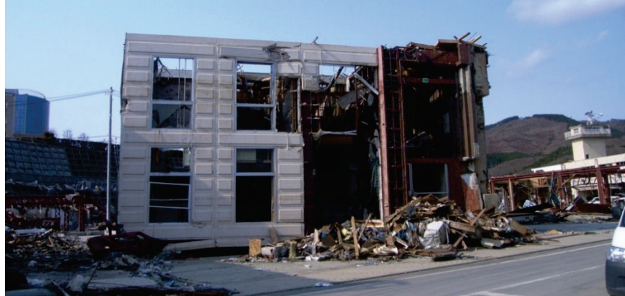
Figure 2-29 Overturned steel-frame office building in Onagawa, Japan, 2011 Tohoku tsunami (photo courtesy of G. Chock and ASCE, from Chock, et al., 2013b).
