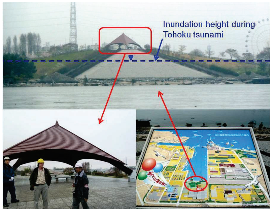
Figure 4-1 Soil berm in a community park at the Port of Sendai, Japan. Concrete lining on the ocean face deflects incoming waves while sloped sides allow easy access. Map inset identifies the location of berm within the Port (images courtesy of I. Robertson and ASCE, from Chock, et al., 2013b).
