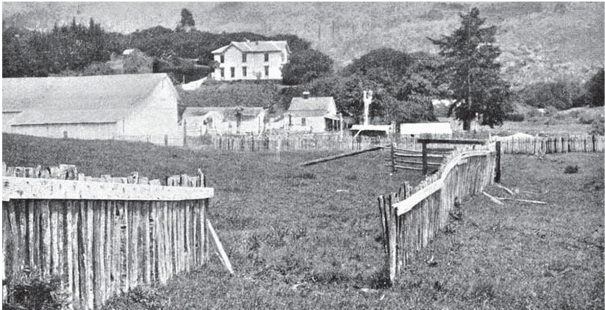
Figure 1-14 Horizontal offset of a fence near Point Reyes, California from fault rupture in the 1906 7.8M San Francisco Earthquake (from USGS).
