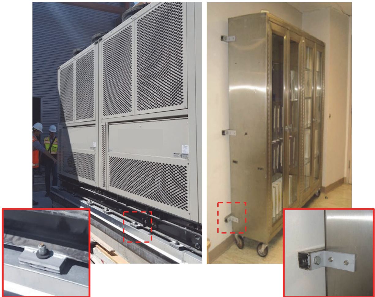
Figure 9-1 Examples of nonstructural anchorage. Left: Rooftop air handler anchored to a housekeeping pad. Right: Shelving unit mounted to a wall (from FEMA E-74).
