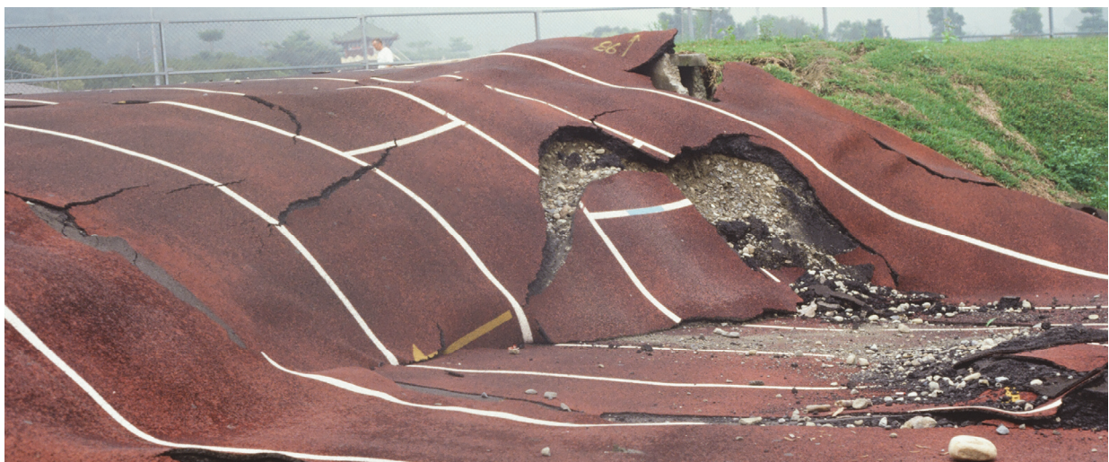
Figure 1-15 Vertical fault offset of a school track from surface fault rupture in the 1999 M7.7 Chi-Chi Earthquake in Taiwan (from B. Yeats).
