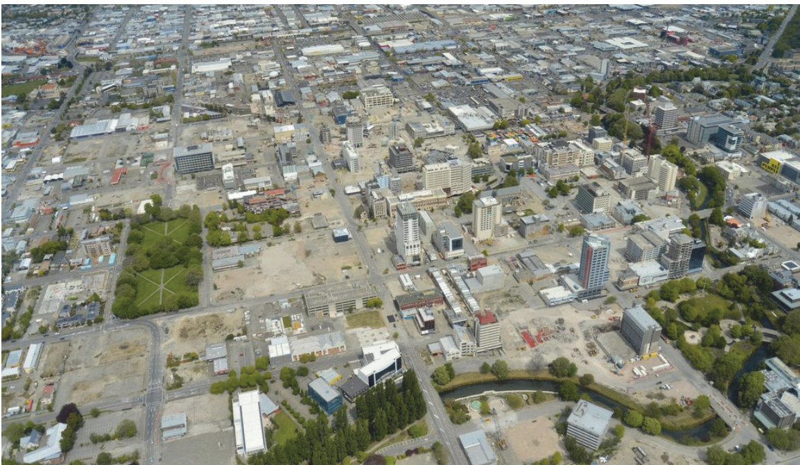
Figure 3-2 Christchurch, New Zealand after demolition of many buildings in the Central Business District following the 2011 Christchurch Earthquake (from Miyamoto International).
