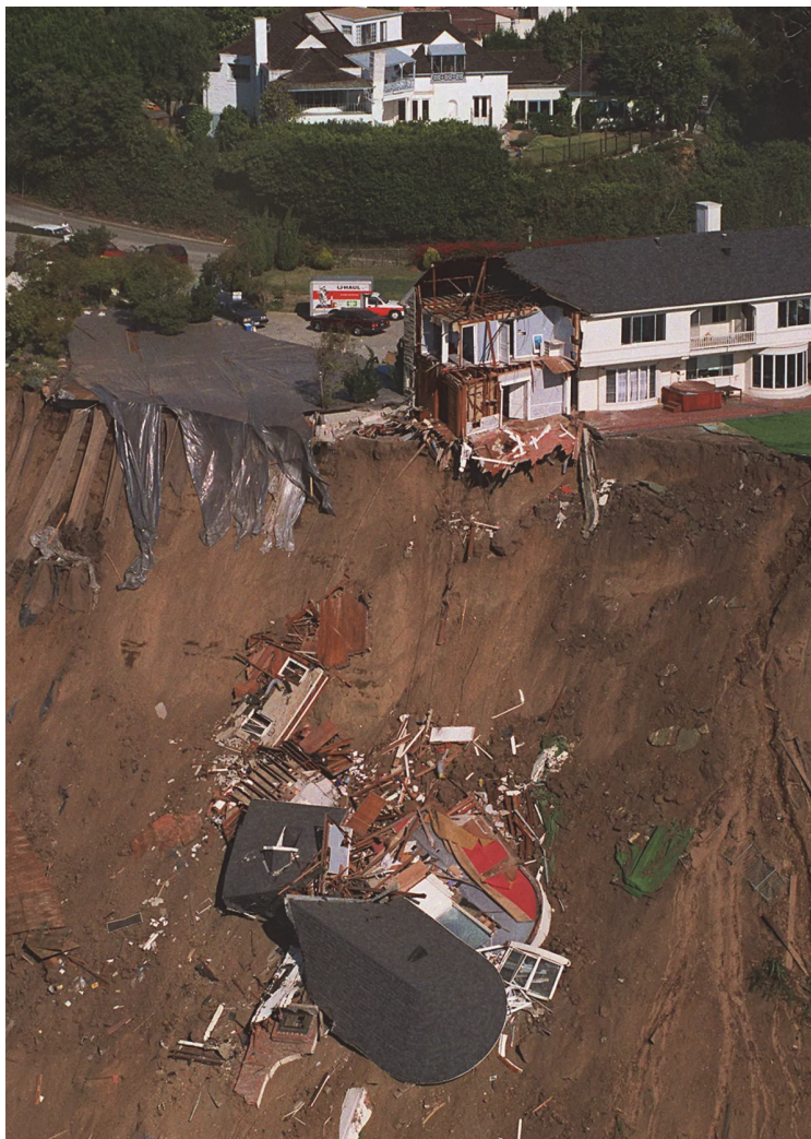
Figure 1-10 House destroyed when the hillside beneath it gave way following the 1994 M6.7 Northridge Earthquake (from Douglas C. Pizac/Associated Press).
