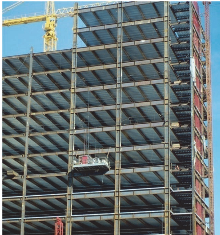
Figure 5-9 A tall steel moment frame structure under construction.
