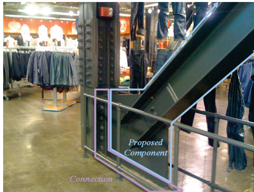
Figure 3-11 Illustration of proposed component and connection definitions for a steel concentrically braced seismic-force-resisting system.
