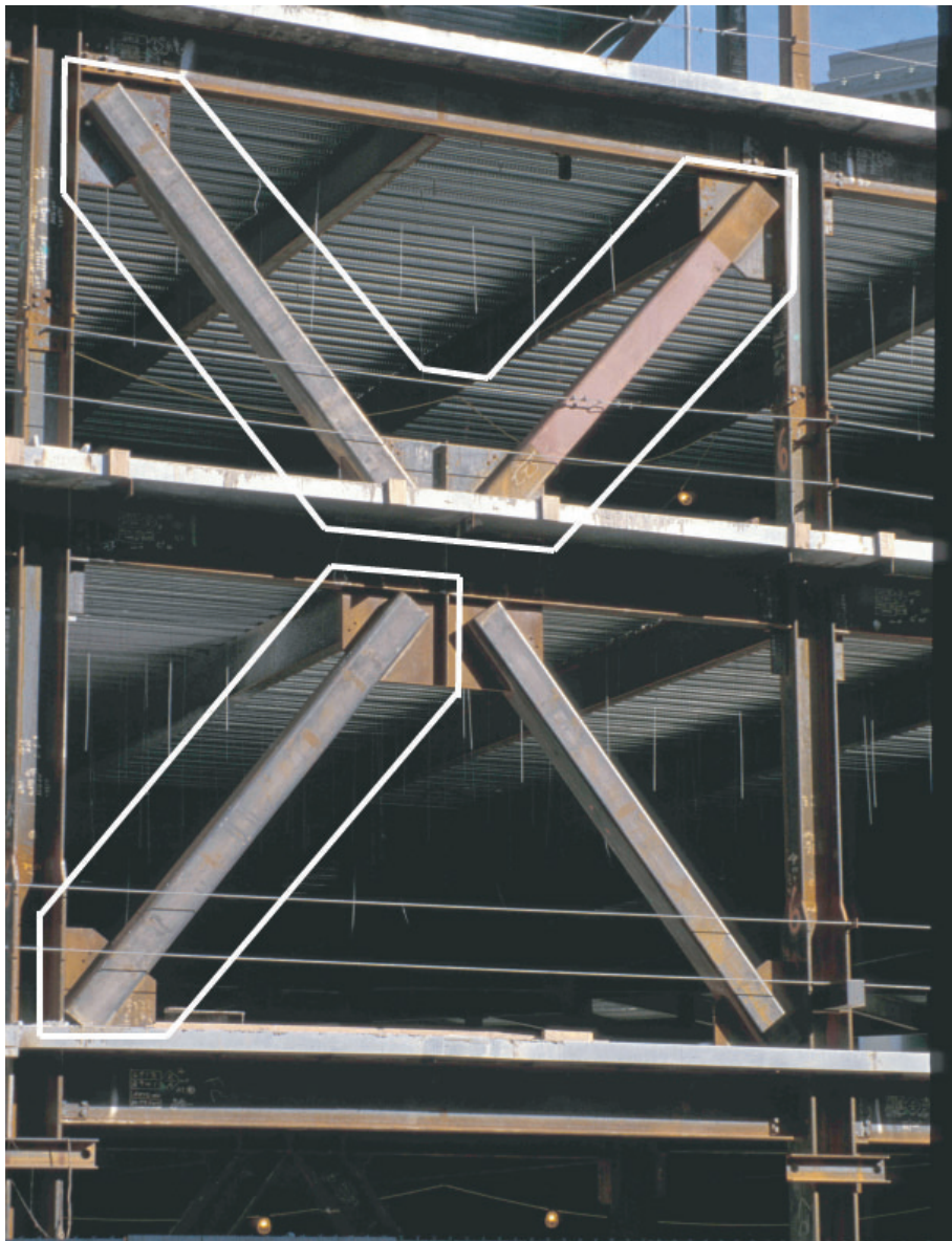
Figure 3-12 Illustration of two alternative definitions for the proposed component boundary in a steel concentrically braced seismic-force-resisting system (Engelhardt, 2007).
