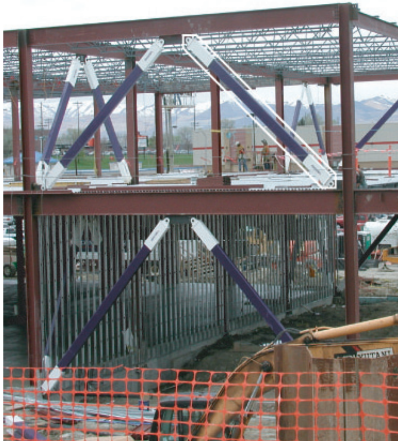
Figure 3-13 Illustration of the proposed component boundary for a buckling-restrained brace seismic-force-resisting system (Engelhardt, 2007).
