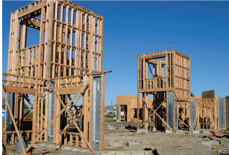
Figure F-1 Example residential building application of high-aspect ratio pre-fabricated wall components ( www.sbebuilders.com/images/hardy-frame-2.jpg ).
