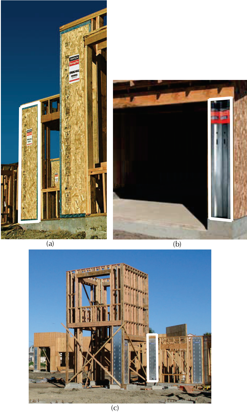
Figure 3-14 Illustration of proposed component boundaries for various wood light-frame shear walls, including (a) Simpson Strong-Tie (2009), (b) Simpson Steel Strong-Wall (Photo courtesy of Tools of the Trade Magazine, 2006), and (c) Hardy frame (Photo courtesy of SBE Builders).
