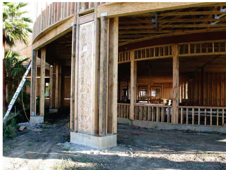
Figure F-2 Example commercial building application of high-aspect ratio, pre-fabricated wall components ( www.sbebuilders.com/images/strong-wall.jpg )
