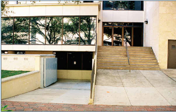
Figure 3-23. Flood doors incorporated into the existing building façade (source: Walter P. Moore)
