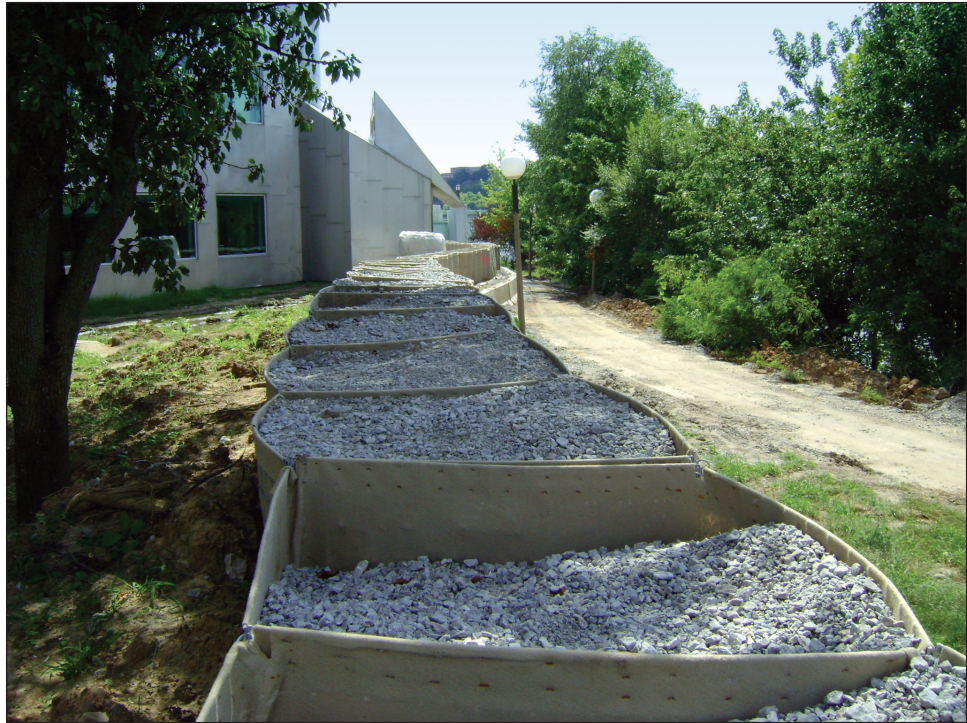
Figure 4-24. Gravel-filled containers that formed a barrier to protect the University of Iowa (2008)
