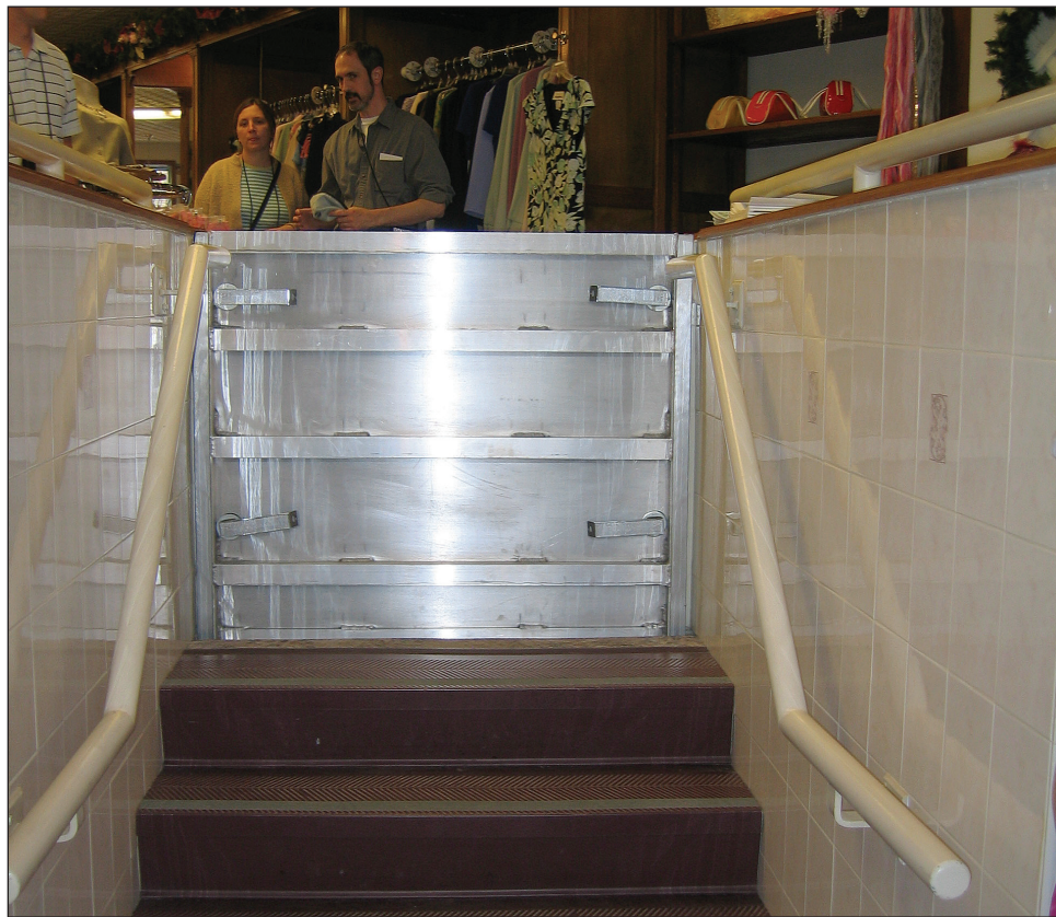
Figure 4-28. Commercial structure in Darlington, WI, mitigated using a combination of wet and dry floodproofing techniques
